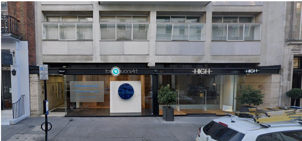
Figure 1: Existing shopfront to number 46 (left), and number 45 (to be mirrored by current proposal)
