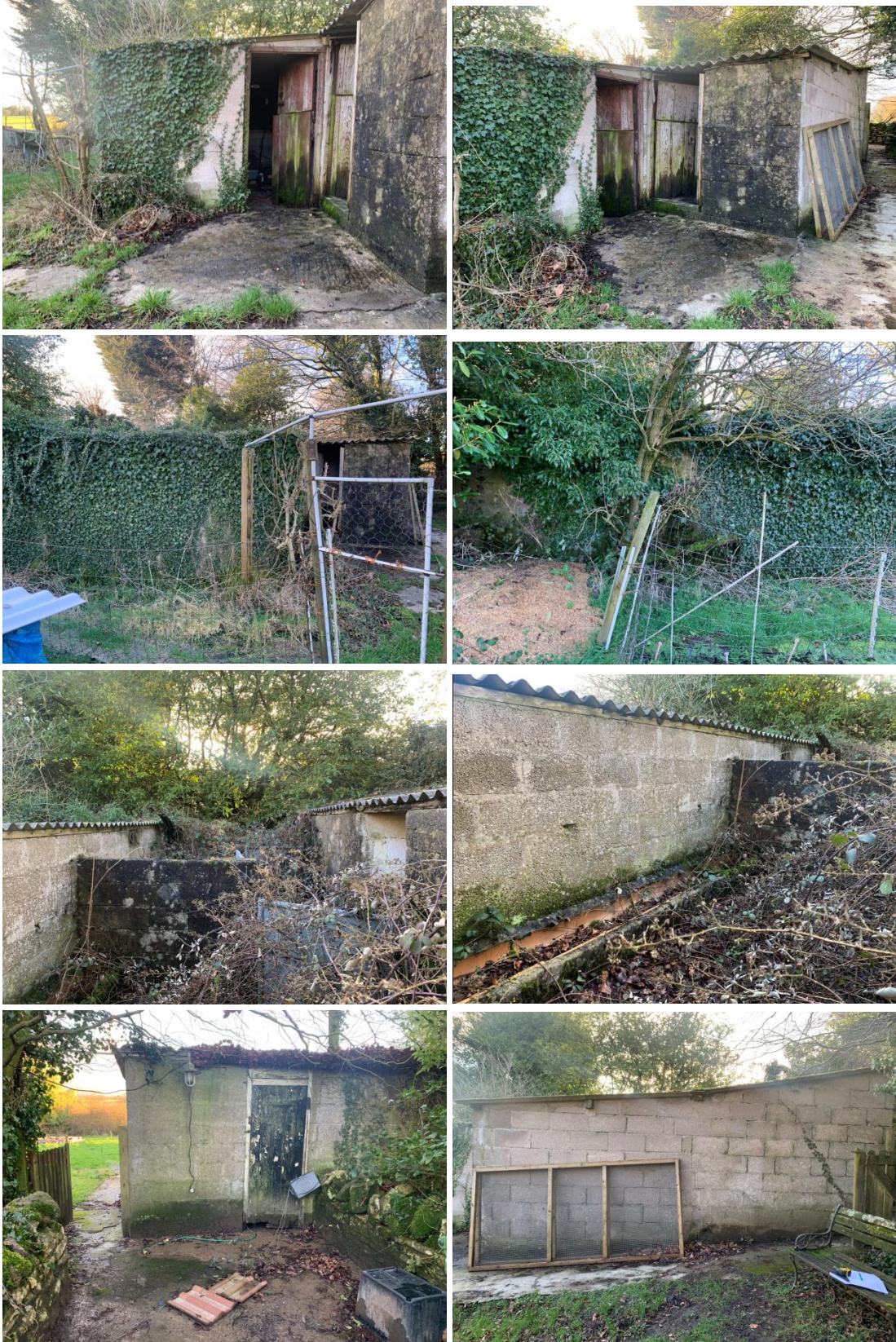
Photos of the Existing Building
