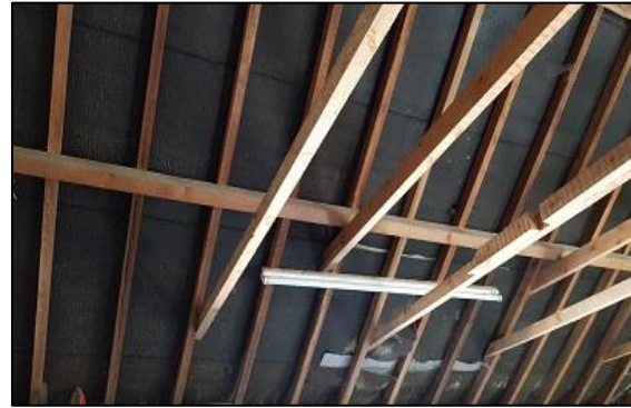
Figure 8: Narrow, machine cut beams.
