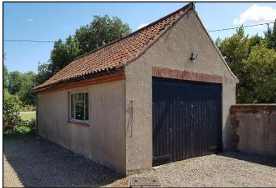
Figure 1: The garage at Church Cottage (western and northern aspect).
