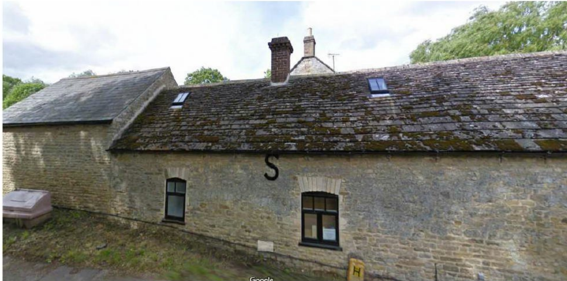
Figure 32 – Examples of Conservation Rooflights within Bulwick
