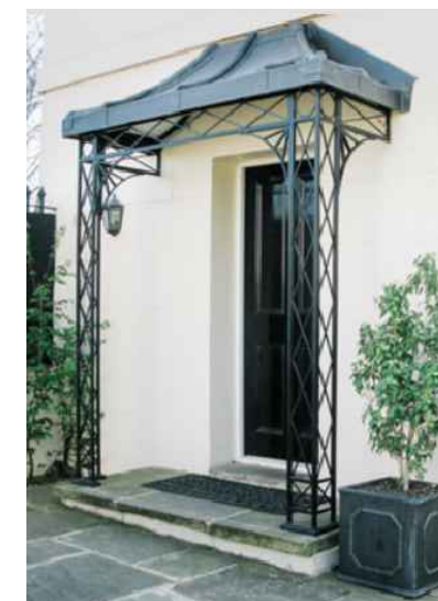
15 - CAST IRON PORCH WITH LEAD ROOF
