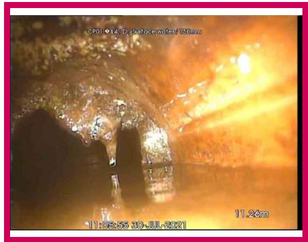
2, 00:00:58, 11.26 m Settled deposits, hard or compacted at joint, 25% cross-sectional area loss
