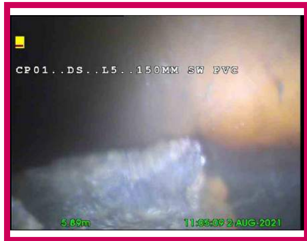
2, 00:01:15, 5.87 m Settled deposits, coarse, 20% cross-sectional area loss, start
