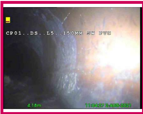
1, 00:00:34, 4.18 m Settled deposits, coarse, 20% cross-sectional area loss
