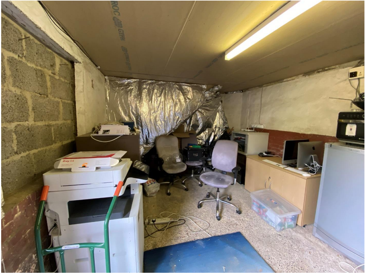
Existing internal photo – note blockwork in wall, plasterboard on the ceiling and modern concrete floor
