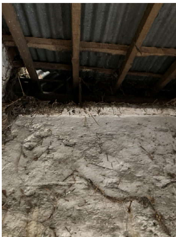
Internal views of cottage 2's external store facing the road. Construction indicates a mixture of block work and cob and stone with a small infilled window evident in the top left hand photograph. Roof comprises a later timber rafter and sheet roofing material.
