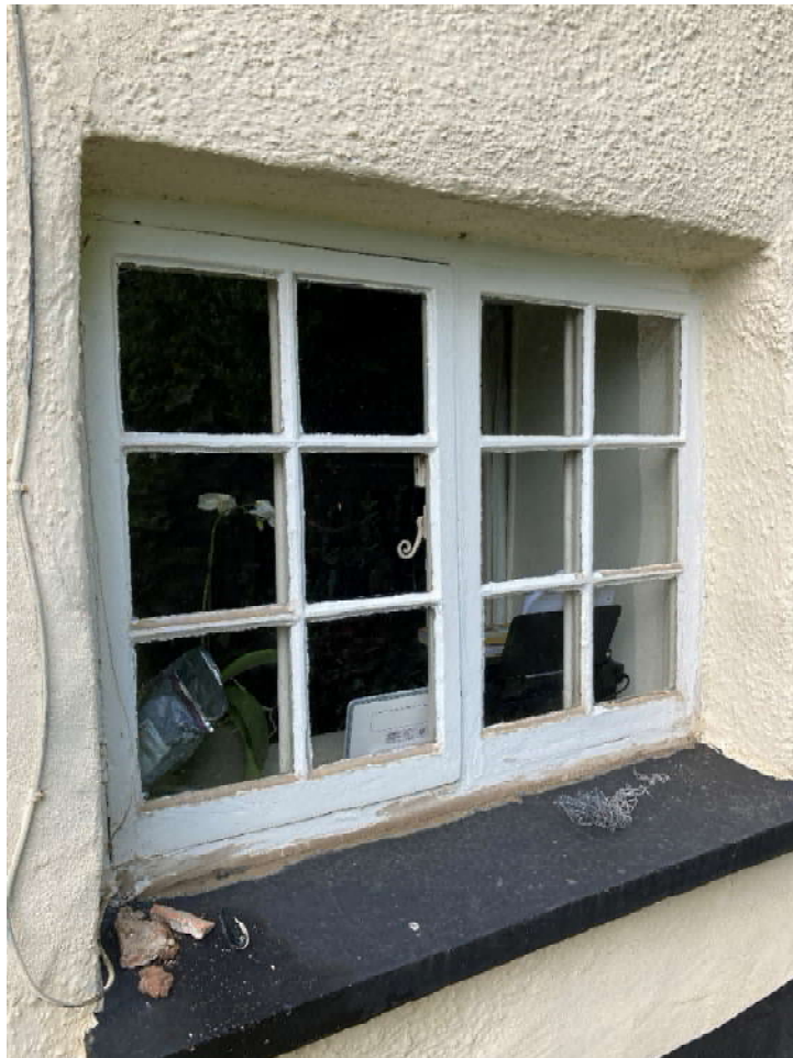
Detail image of typical window on the buildings.
