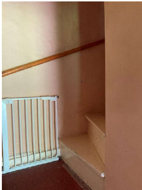
Detail photograph – winding stairs in cottage 1.
