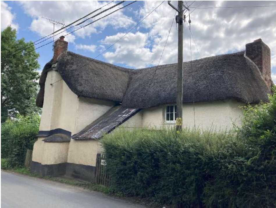
East, road facing elevation. Cottage 1 is on the left and cottage 2 on the right.
