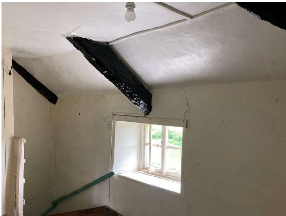
First floor landing, cottage 2.
