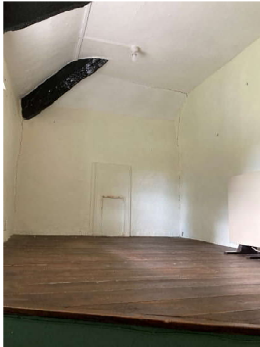
First floor landing, cottage 2 – note small C20 fireplace.
