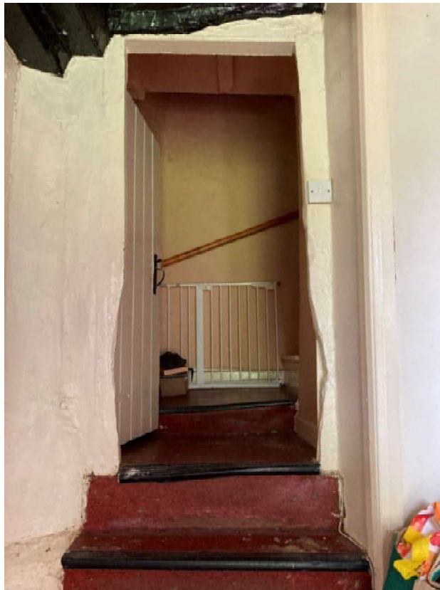
Cottage 1 – View of later opening formed with steps to link cottage 1 and cottage 2.
