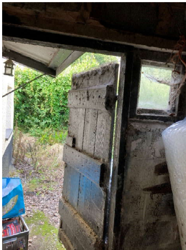
Internal view of East elevation cottage 2 store facing the road.
