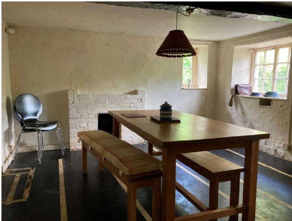
Cottage 2 – Dining area at North end of house. Note later C20 brick fireplace.
