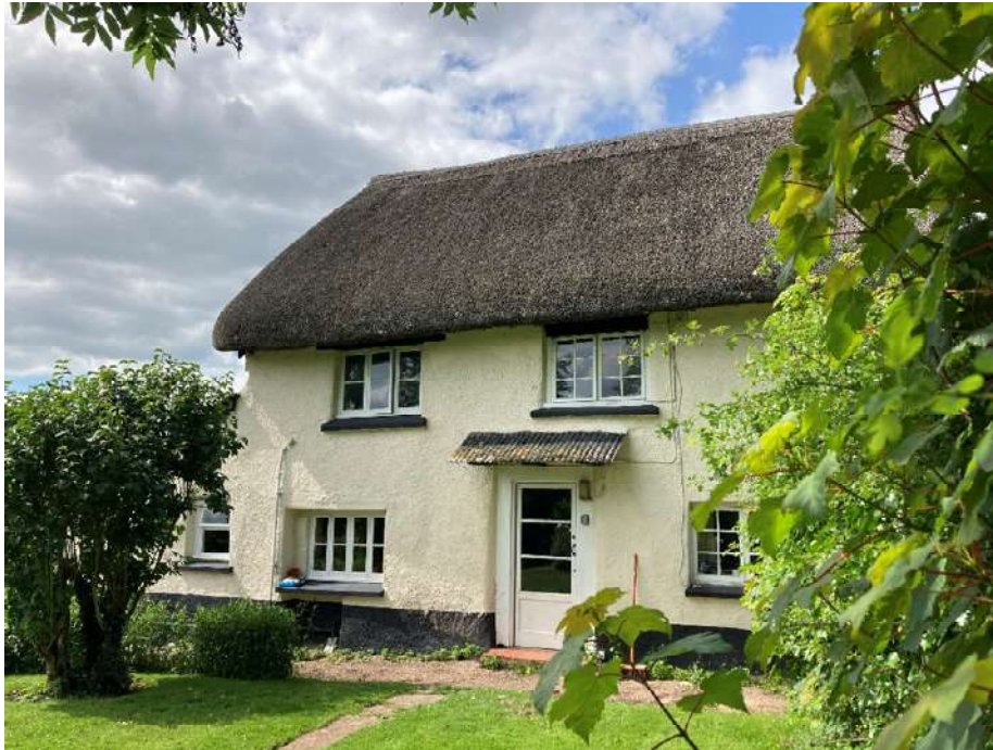
South facing elevation of cottage 1 showing front door.
