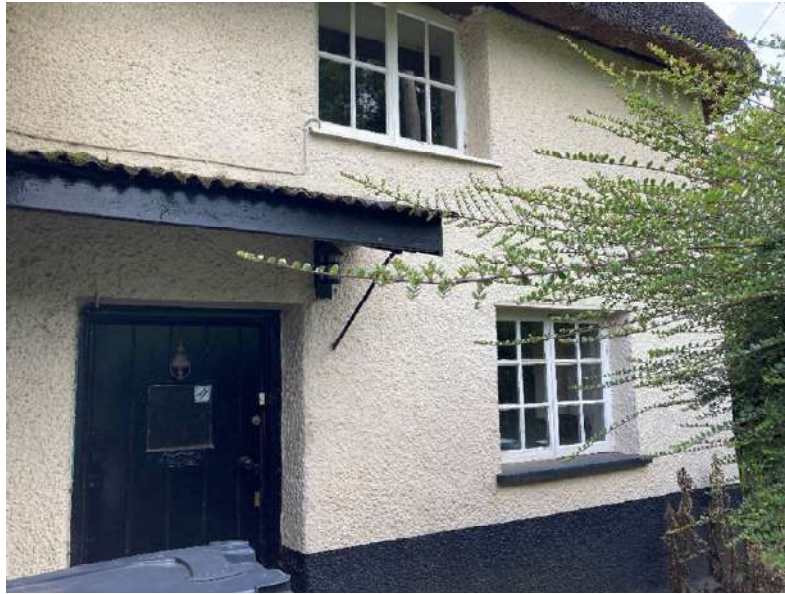
Detail view of cottage 1's front door and porch.
