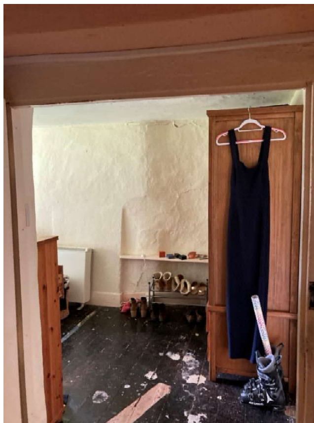
First floor bedroom, cottage 1 – note chimney breast and infilled fireplace.
