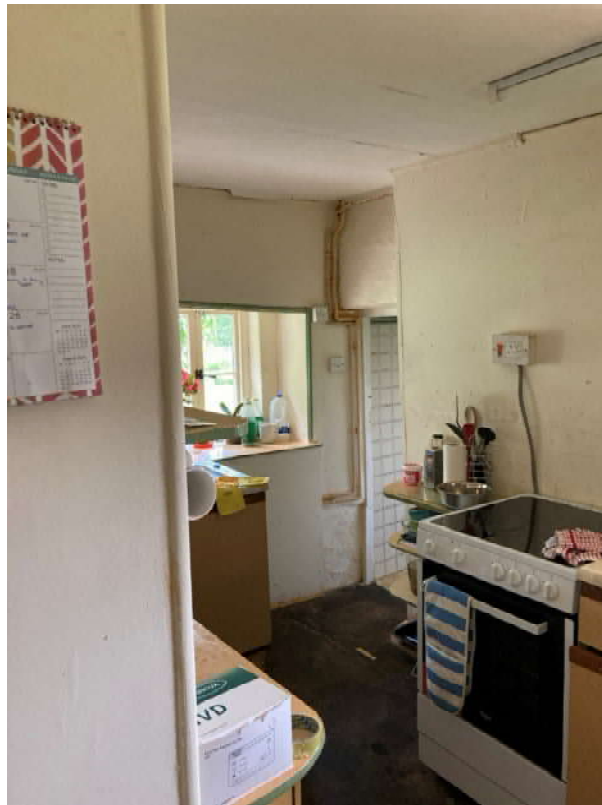
Cottage 1 – C20 (circa. 1970's) kitchen installed in original hallway.
