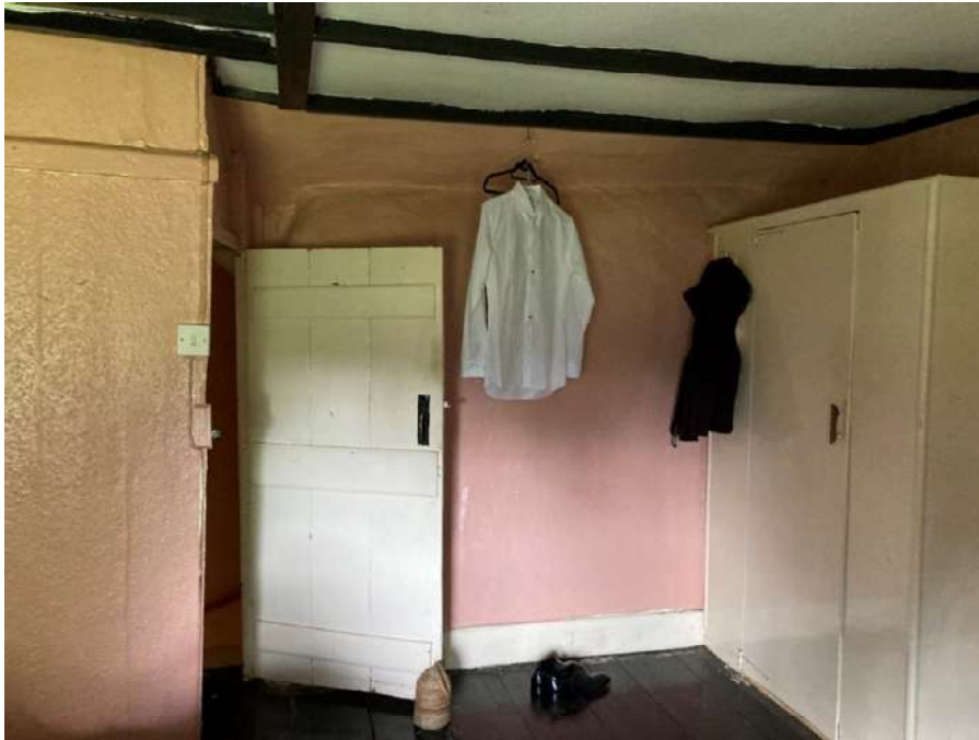
First floor bedroom, cottage 1 – note original door and ceiling beams.
