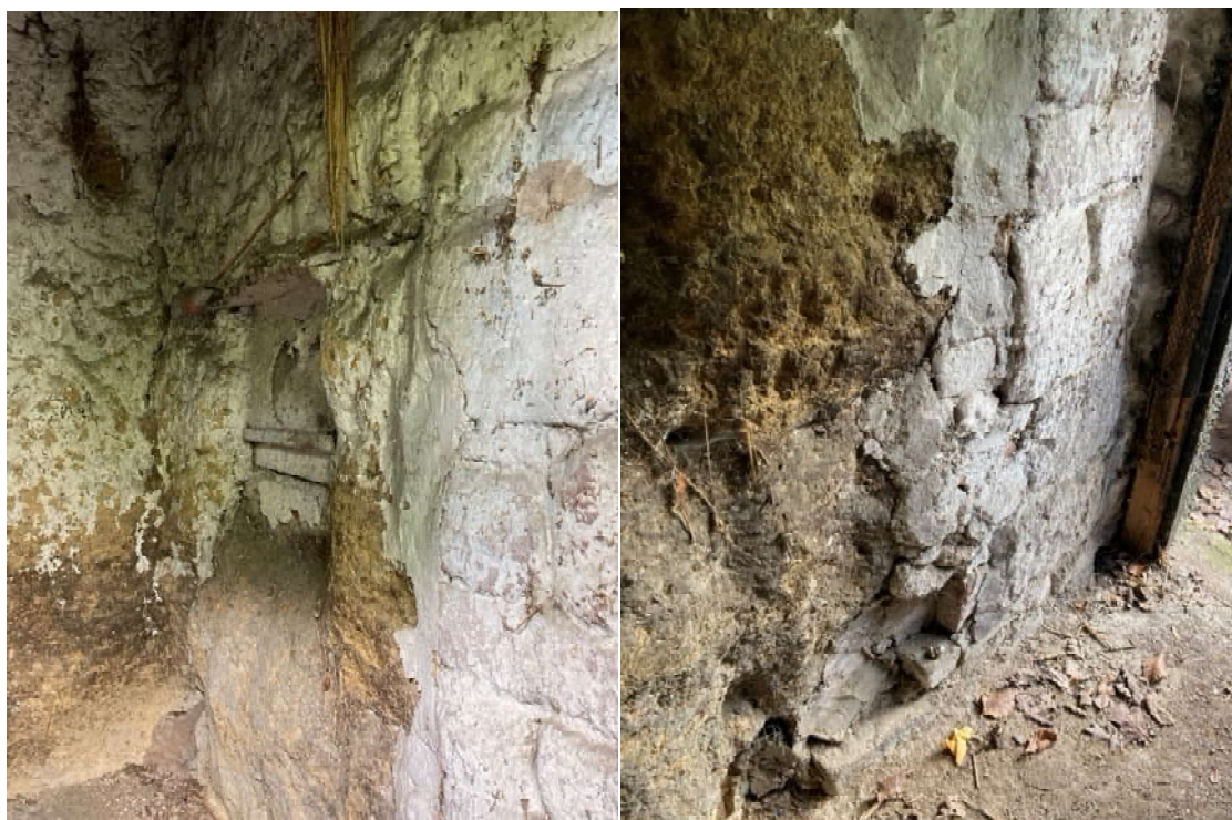
Internal views of cottage 2's external store facing the road. Construction indicates a mixture of block work and cob and stone with a small infilled window evident in the top left hand photograph. Roof comprises a later timber rafter and sheet roofing material.
