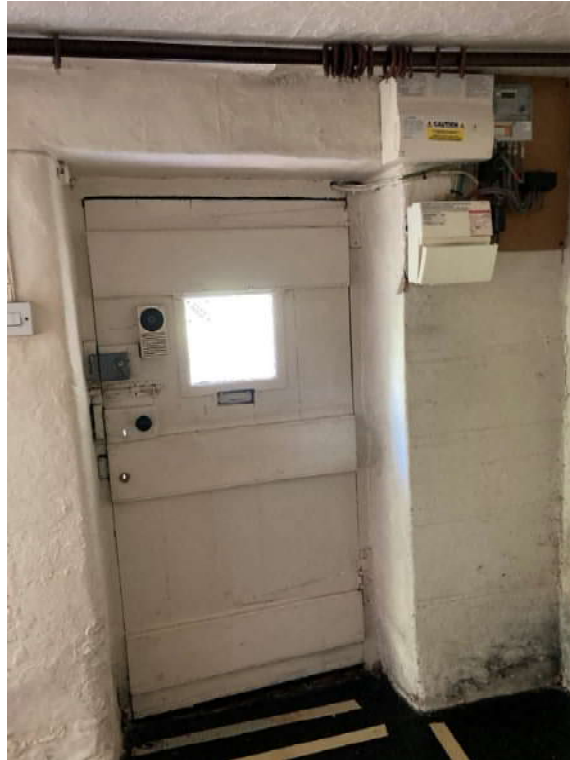
Cottage 2 – Road facing entrance door.
