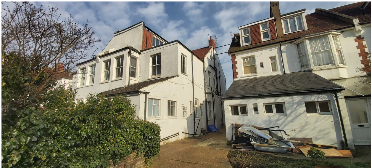
Figure 2 – Rear Elevation of the existing building on the left, with gabled tile roof and white painted walls.
