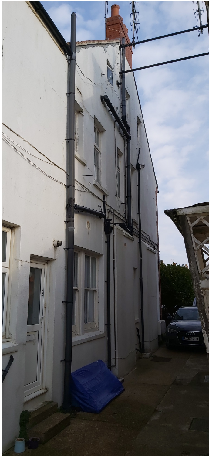
Figure 4 – Photo of side elevation with uPVC door and window to be blocked up
