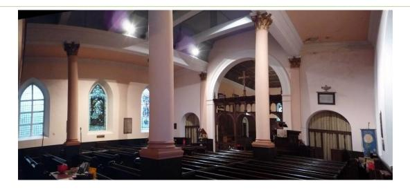
Interior: each aisle has 2 unfluted Corinthian columns on tall bases; C19 wood west gallery. Coved ceiling with exposed tie beams. Semi-circular chancel arch with smaller similar flanking openings; early C20 screen incorporating early C18 carved woodwork with flower and leaf motifs; encaustic-tiled chancel floor and coved, panelled, painted ceiling of 1896.
