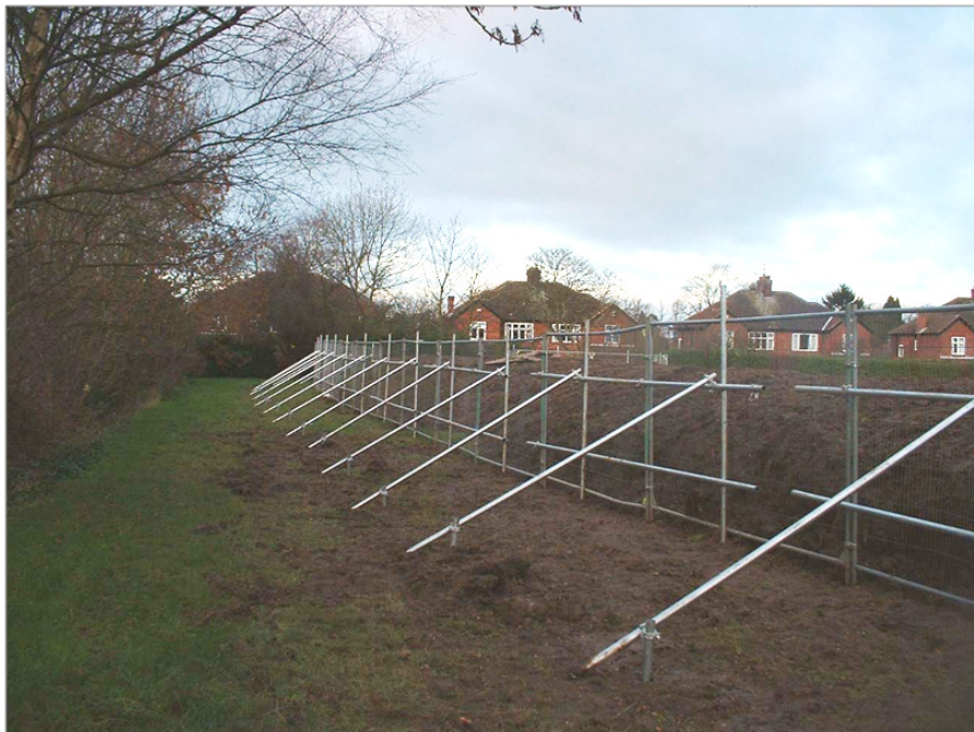
Figure 5 - Example of a barrier erected on a site
