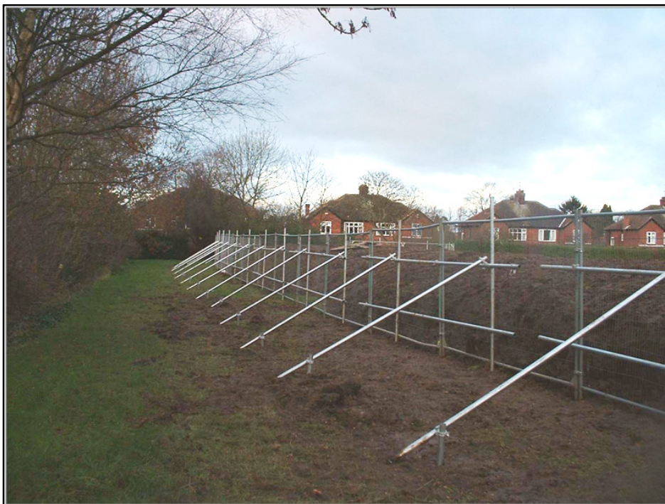
Figure 2- Example of a barrier erected on a site
