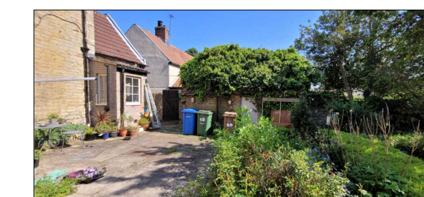
Photo 4 Outbuilding to be demolished
