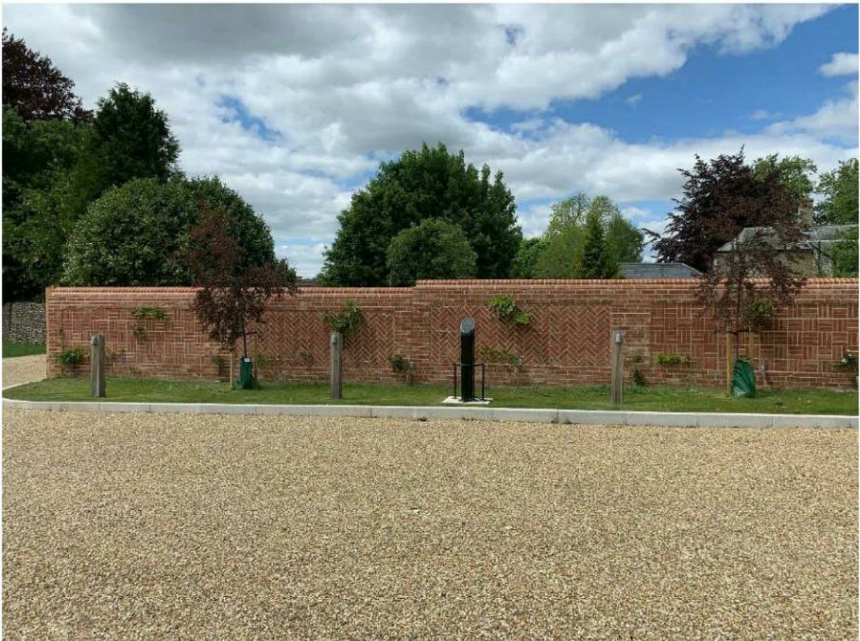
Figure 1: Photograph Image of the existing Wall
