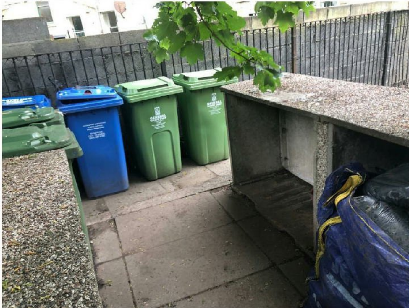
Photograph 2: Existing refuse storage area
