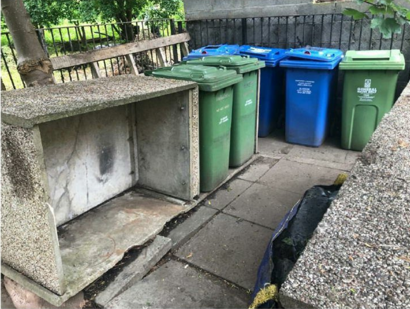
Photograph 1: Existing refuse storage area
