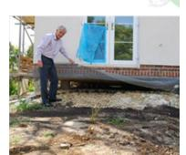
The completed deck with pile overlays made of flexible material prevents concrete from the slab pour leaching onto the ground surface. Similarly the aluminum strips between the sheets of ply prevent concrete reaching the ground surface.
