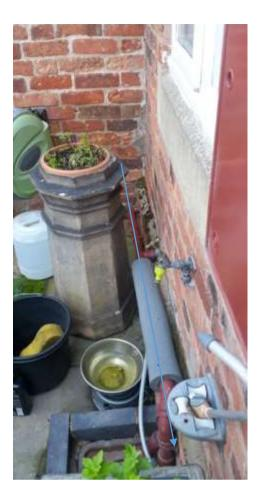
Image 2 – Photo showing location of condensate pipe under kitchen window. Approximate location indicated by the blue line.
