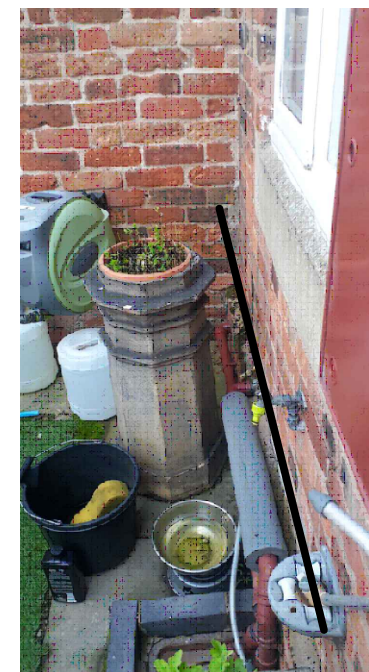
Image 2 – Location of condensate pipe through wall to drain under kitchen window
