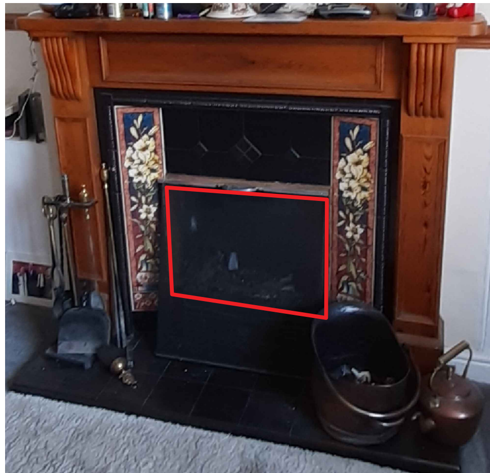
Image 1 – Existing fireplace with back boiler to be decommissioned and stove installed to existing opening. The existing grate and ash pan will be removed and the insert installed to the area shown in red. Note: The NT Vernacular Building Survey indicates that this is a 1970s installation.
