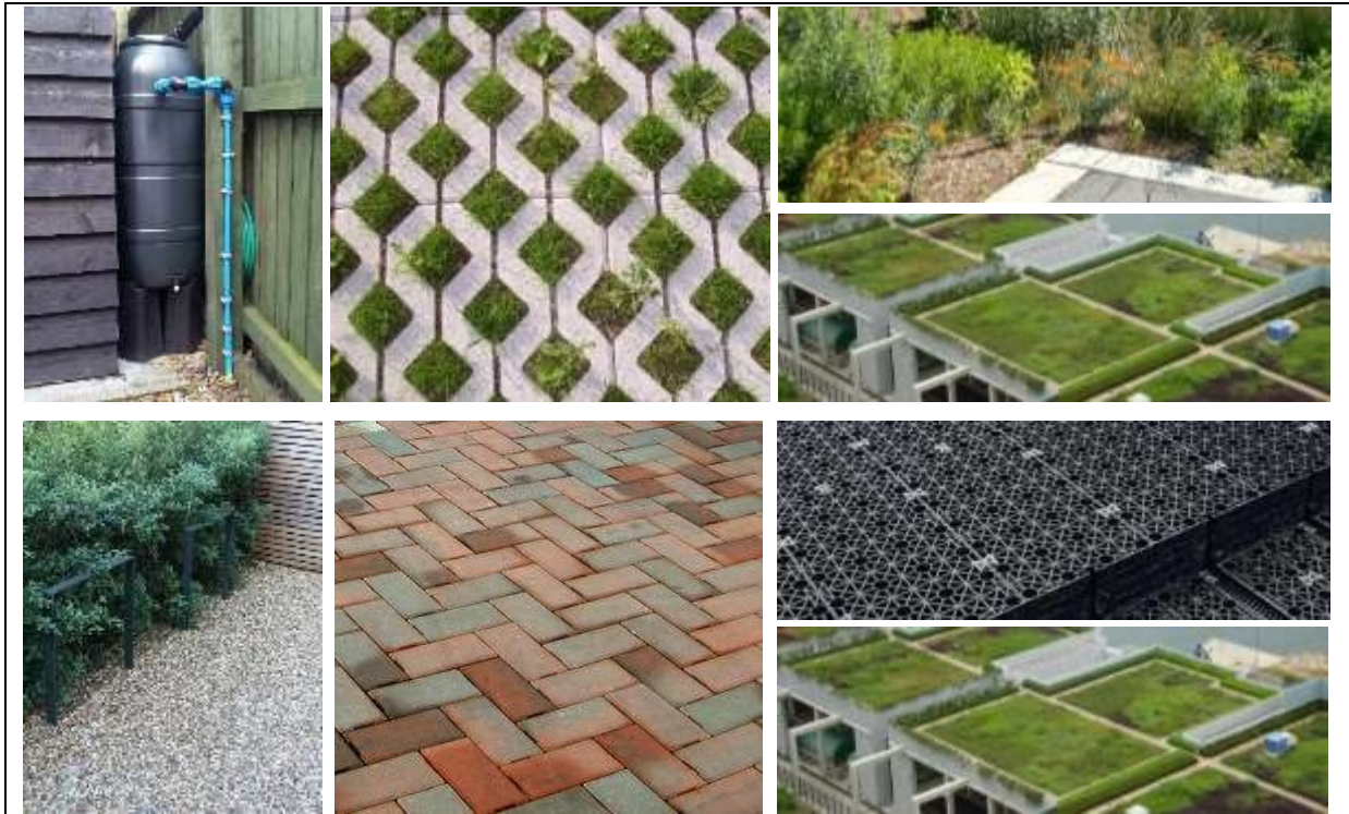
Figure 1: Surface water storage facilities and potential SuDS features - rainwater harvesting, on-site tank storage, rain garden soak-away and green roofs. (Source: UK SuDS Manual)
