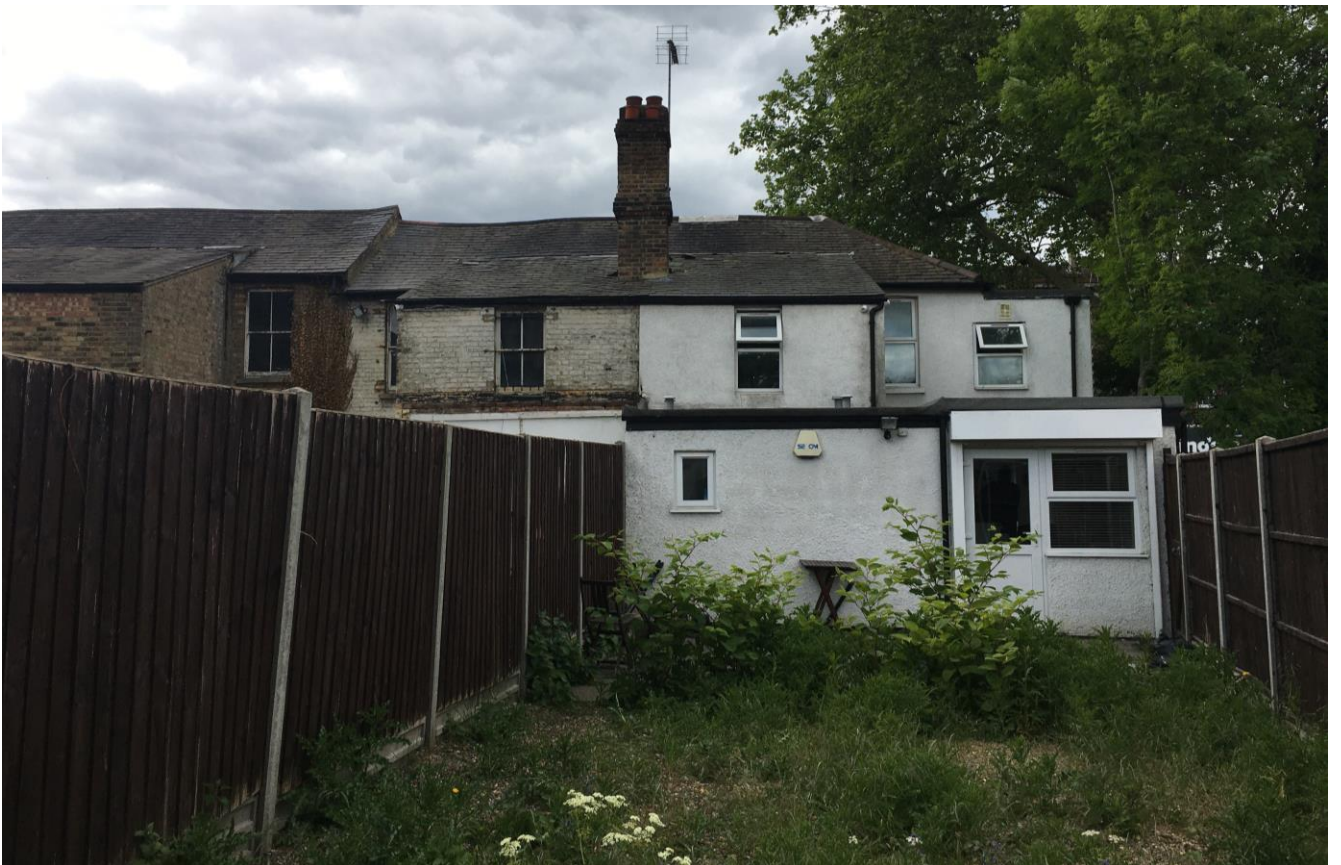
View of rear from east within rear garden
