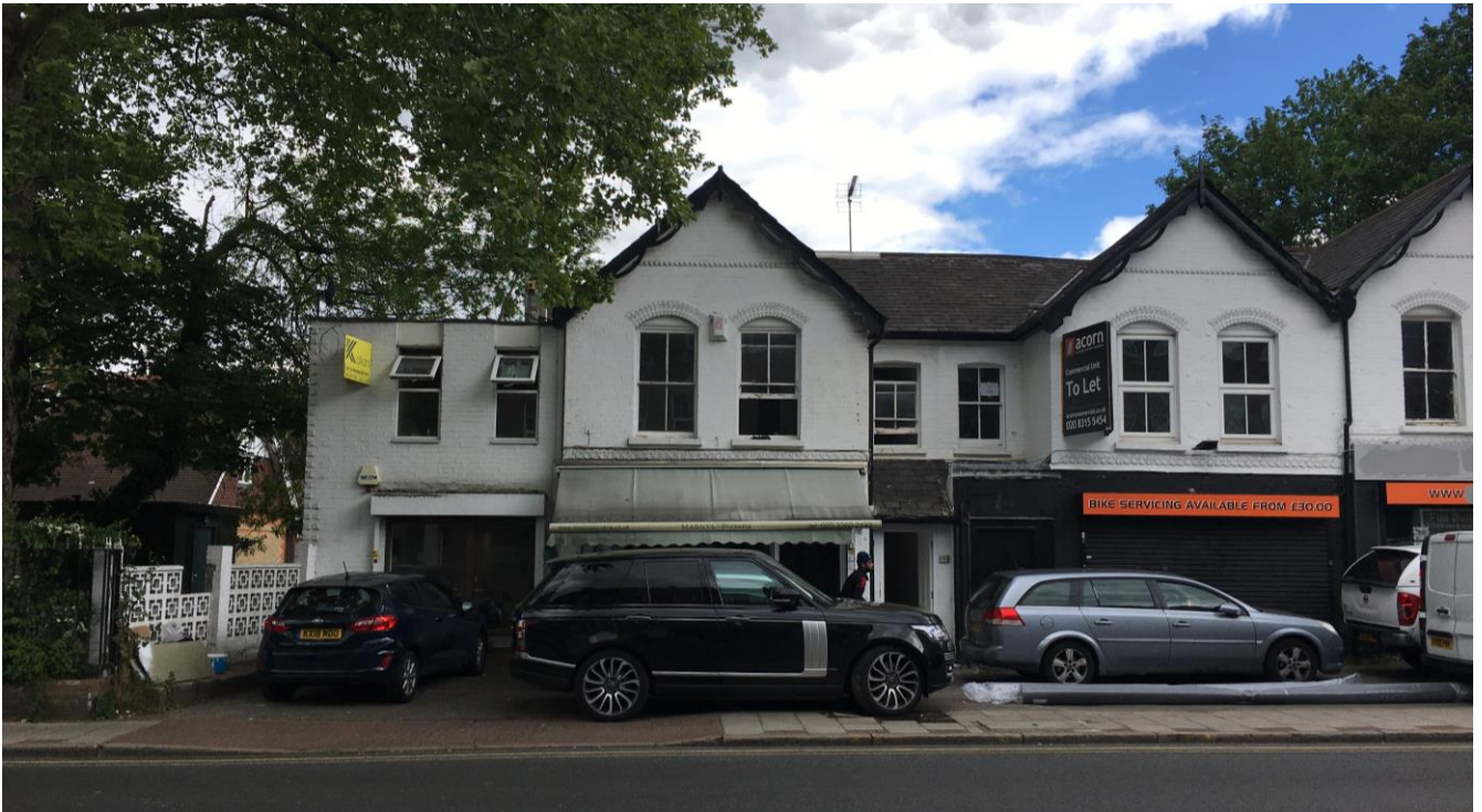
View of front from west on Station Road
