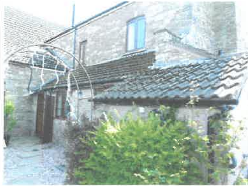
Figure 2 – Sealed roof materials and lead flashing
