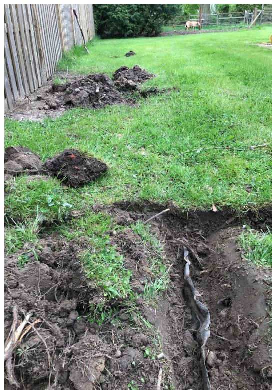
Photo 4 (provided by client): Hand excavations undertaken 05/2021 to show root barrier
