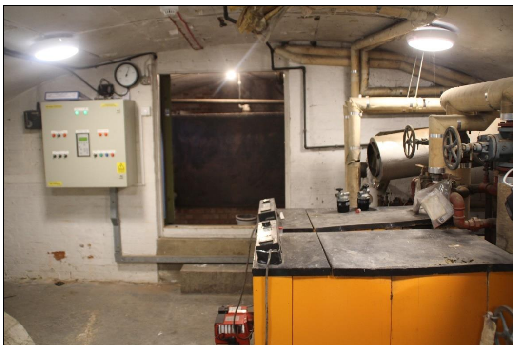
Photo 40. View of the modern brick wall between B3 and B4
