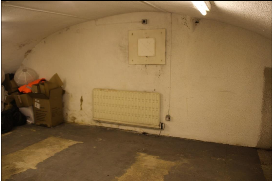
Photo 36. View of Room B2 – arch vaulted cellar
