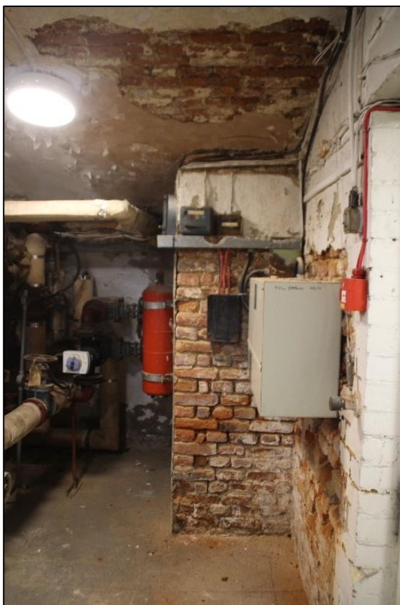
Photo 39. Brick construction of B3
