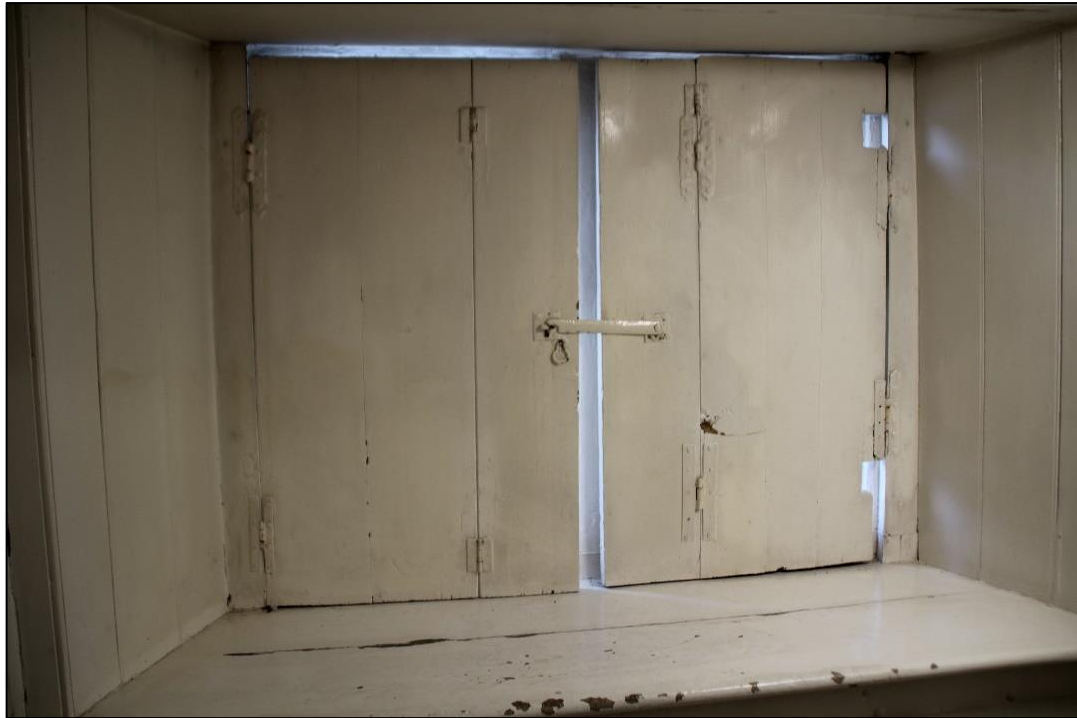
Photo 32. Plank shutters to the small window to the basement stairs, with original ironmongery
