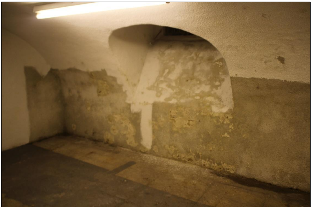
Photo 37. View of blocked window opening in B2
