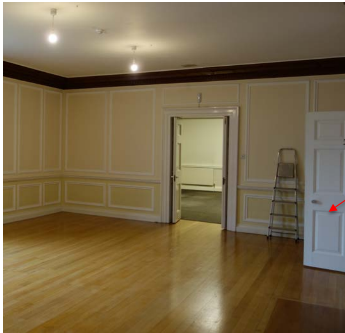
Figure 21 Room D looking towards Room E
