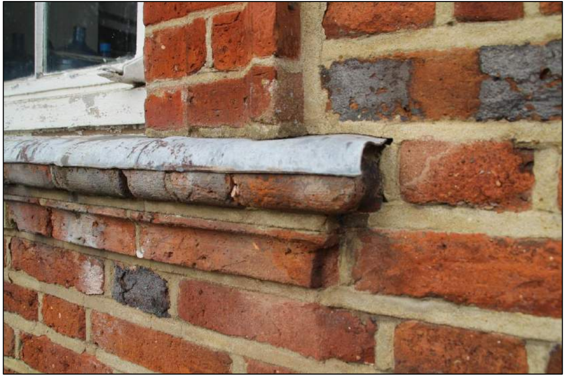
Fig.12 Detail of brickwork, showing gauged brickwork and firing marks
