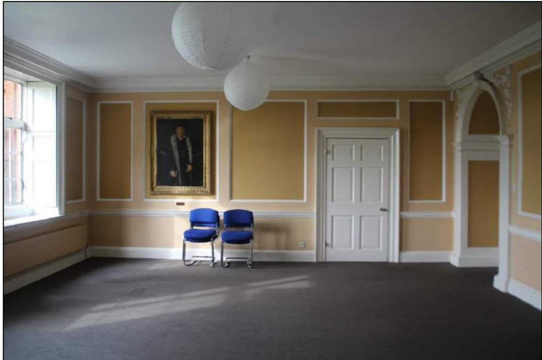
Photo 10. The west wall of Room 3, accessing Room 4
