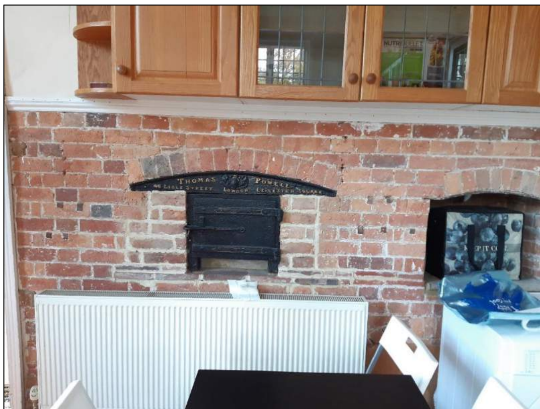
Photo 31a. Former bread ovens in servant's wing
