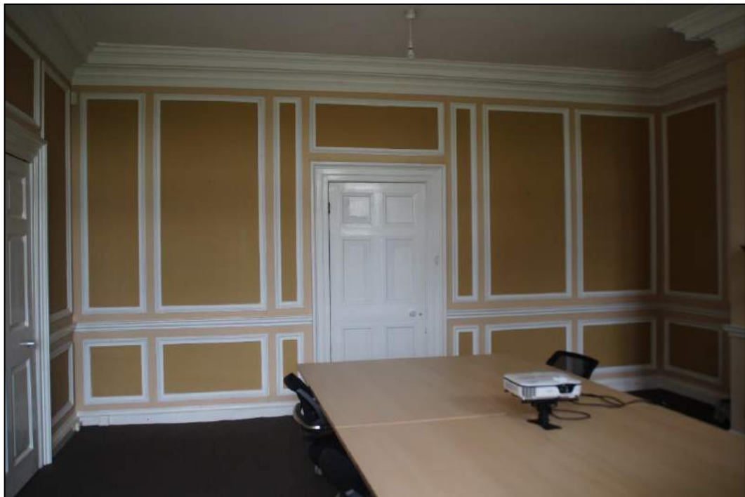
Photo 6. North wall of Room 2 (accessing the entrance hall)
