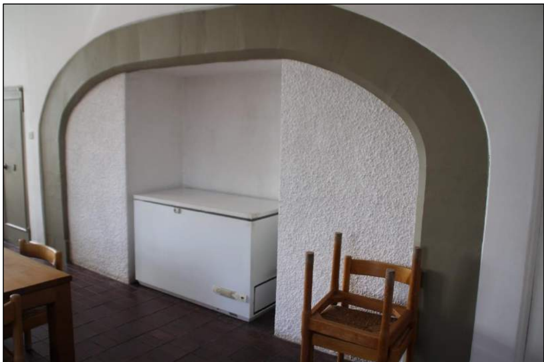
Photo 28. The large stone fire surround which would have housed an open hearth with cooking ranges and equipment
