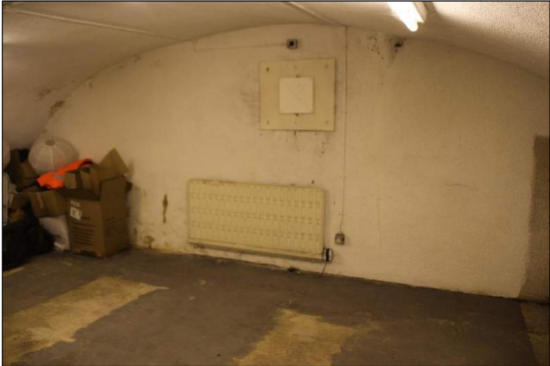
Photo 36. View of Room B2 – arch vaulted cellar
