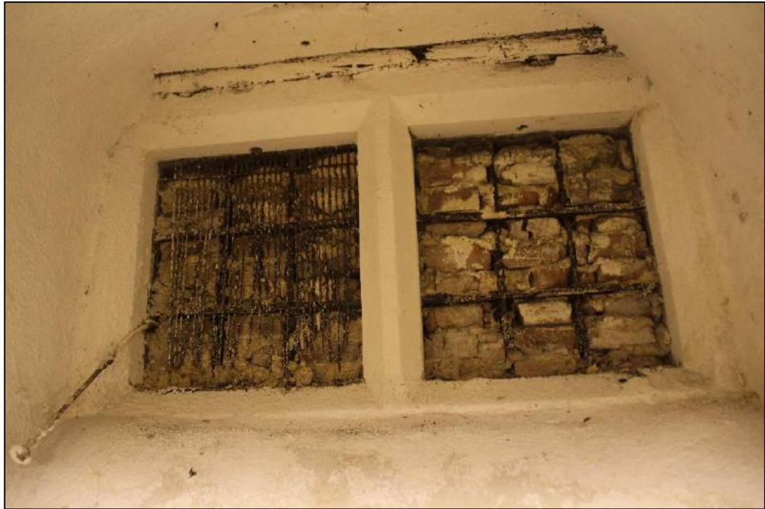
Photo 38. View of blocked mullioned window with iron bars
