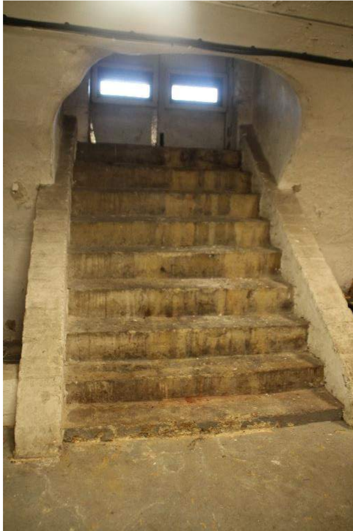
Photo 41. View of steps down from stable courtyard with sloped sides
