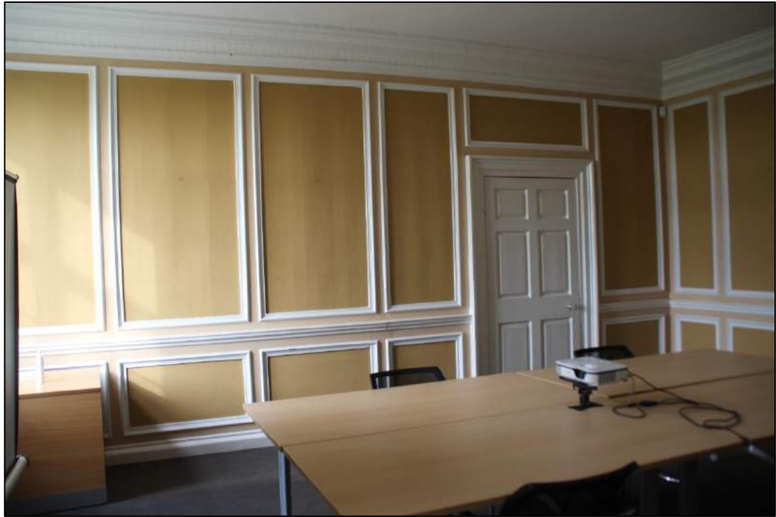
Photo 7. West wall of Room 2, accessing Room 3
