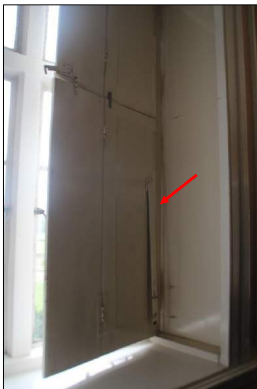
Photo 8. Detail of interior of shutter with long bracket arrowed
