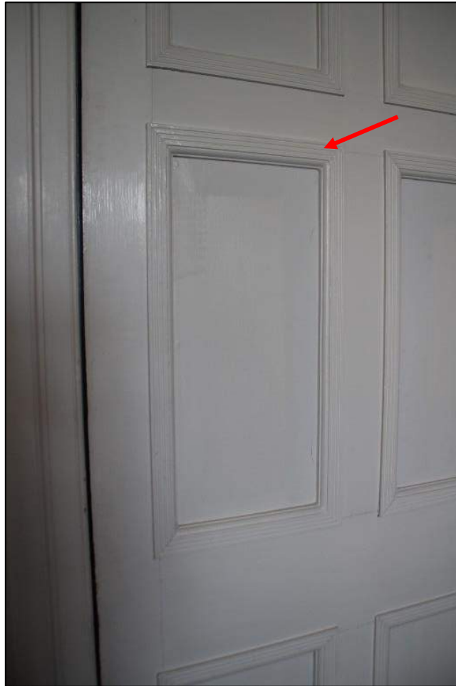
Photo 13 Interesting ridged panel edging on door in Room 3
