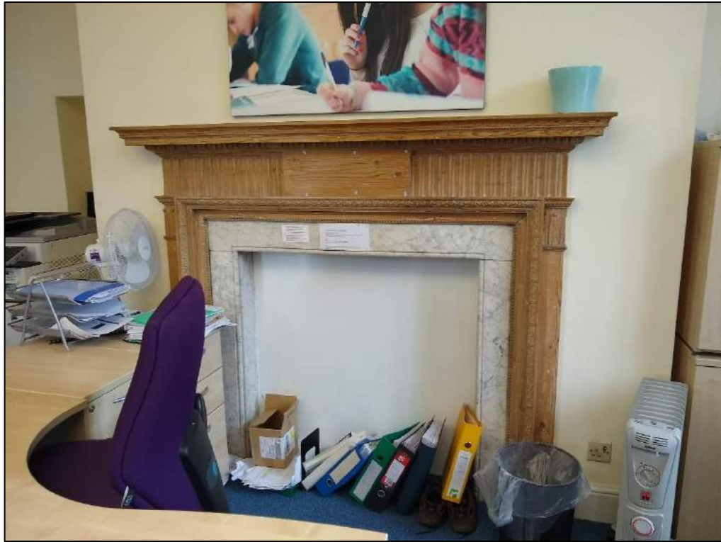
Photo 46. Fireplace in Room 7
