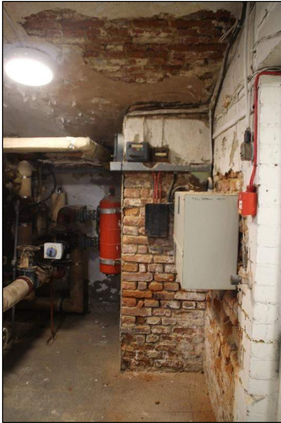
Photo 39. Brick construction of B3
