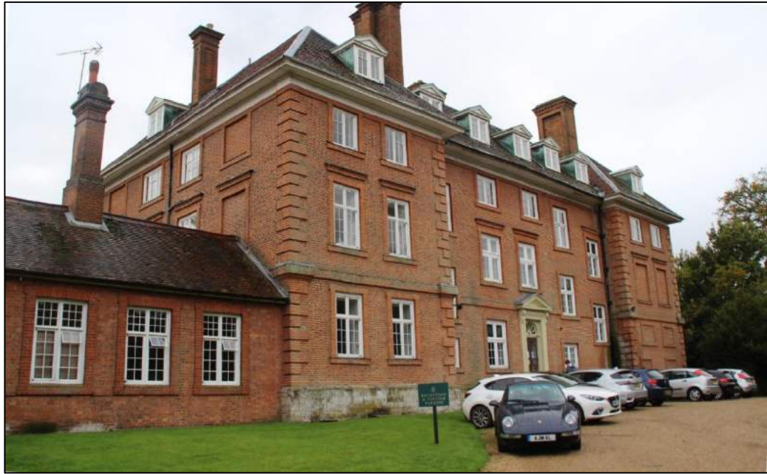
Fig.7 Front (north) elevation of the building
