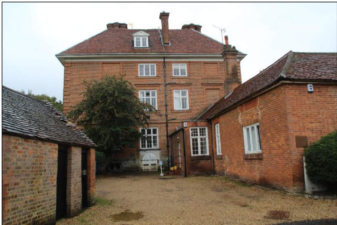
Fig.14 The eastern elevation of the Building, viewed from the stable courtyard
