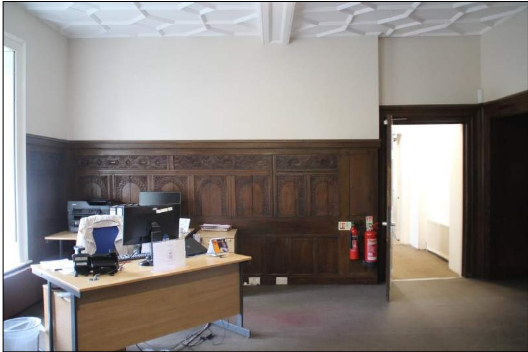
Photo 1. View of the eastern wall of the main entrance hall
