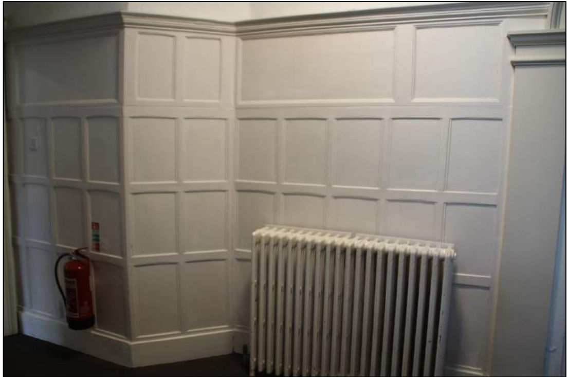
Photo 24. Panelling in the ground floor stair hall
