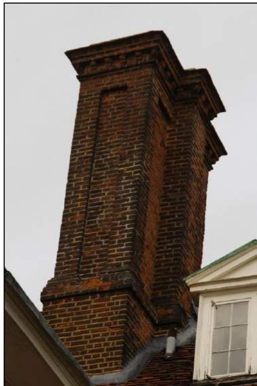
Fig.13 Detail of eastern chimney stack
