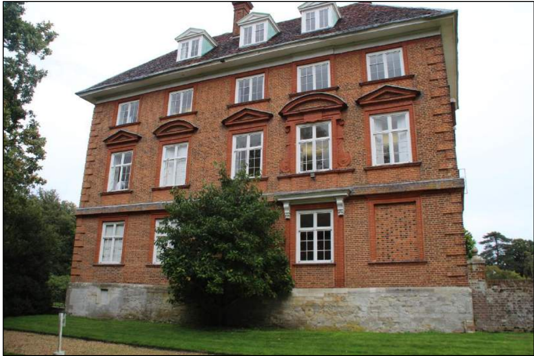
Fig.9 Western elevation, image taken looking east
