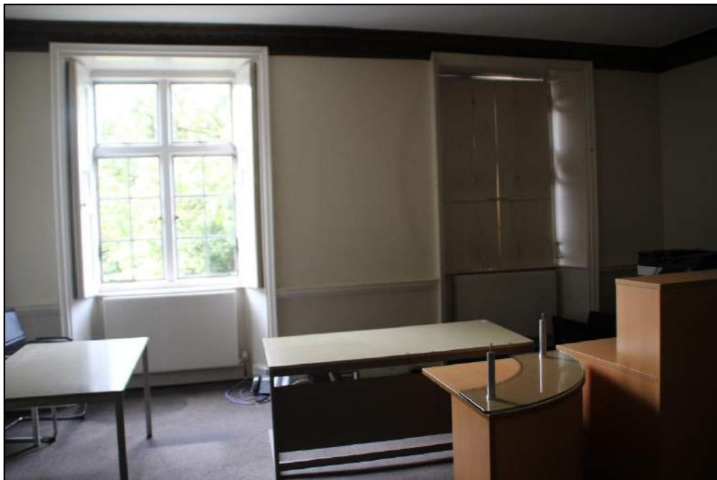
Photo 19. View of the west wall of Room 5
