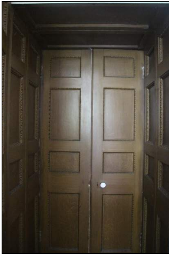
Photo 20. Interior of doors, Room 5 (left)
