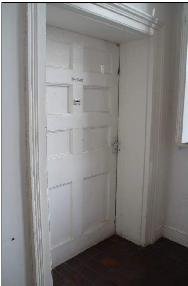
Photo 31 Door to 19th century servant's wing
