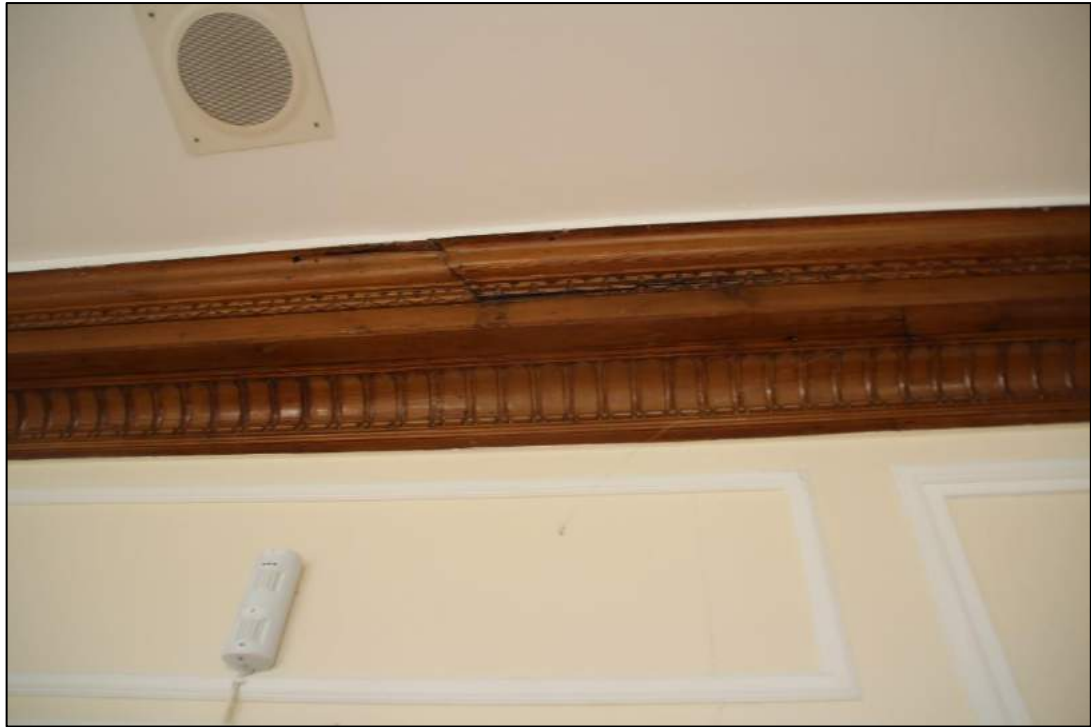
Photo 16. The timber cornice of Room 4
