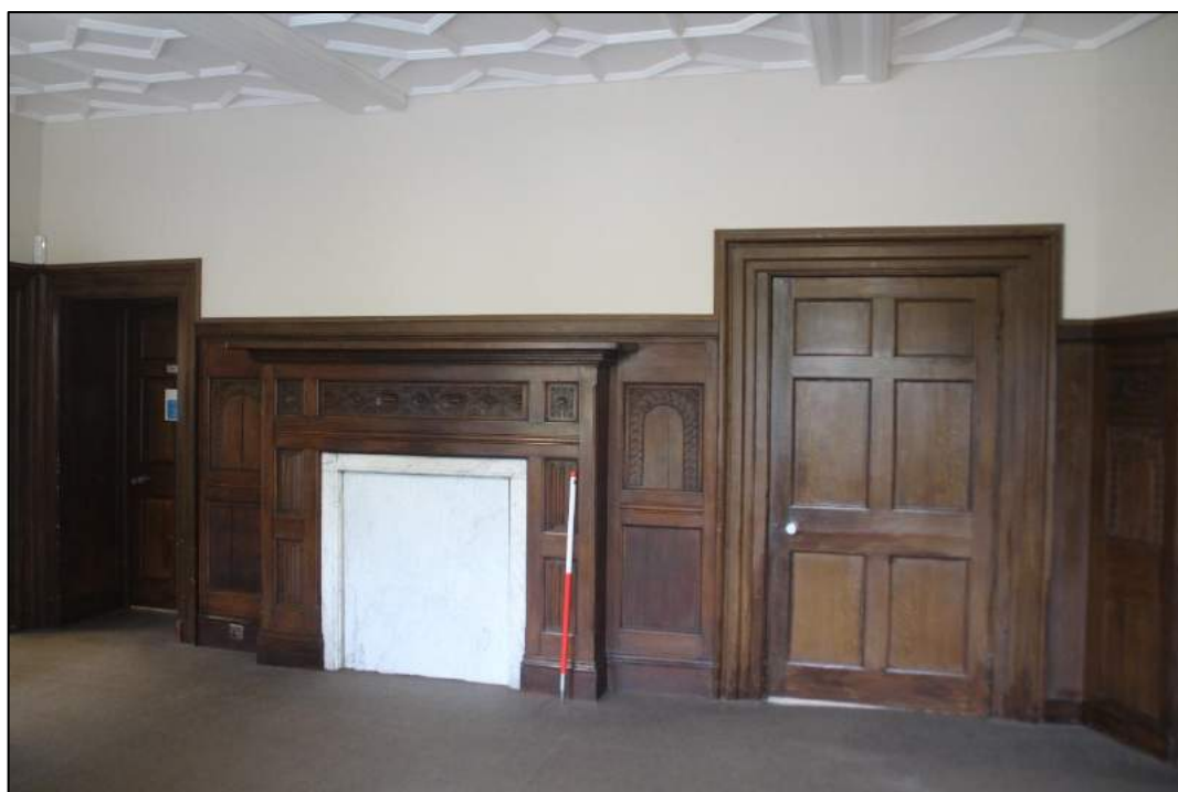
Photo 3. Southern wall of main entrance hall, image looking south
