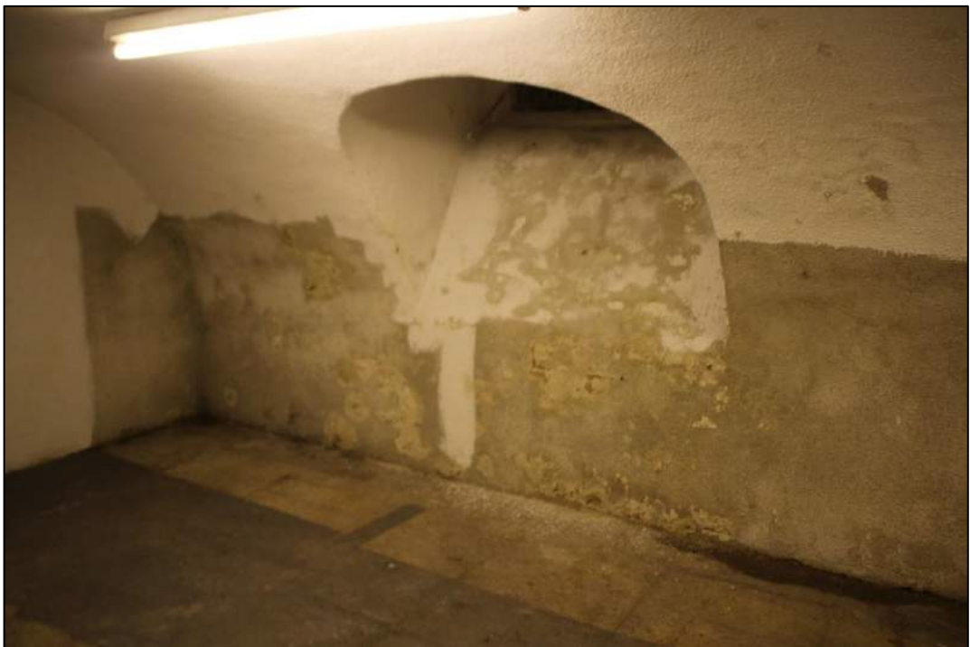
Photo 37. View of blocked window opening in B2
