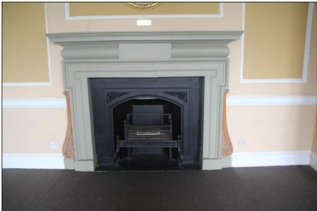
Photo 11. The mantelpiece of Room 3, thought to be original or early 18th century
