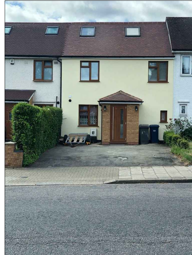
FRONT VIEW OF 13 KINGSBURY ROAD
