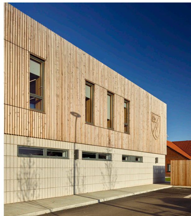
Windows openings and timber cladding
