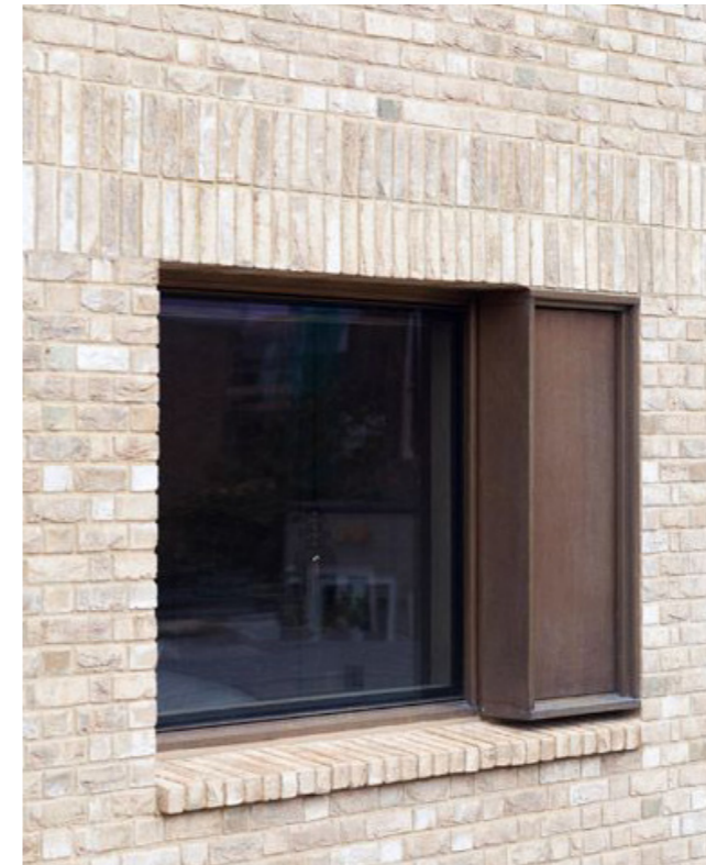
Soldier Course Brickwork
