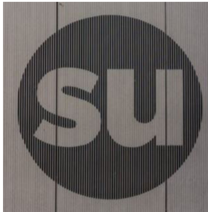
Signage within the cladding
