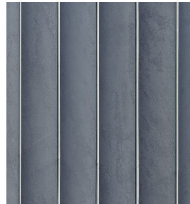
Vertical Fins within Cement Board Cladding
