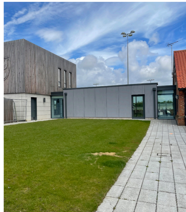
Cement Board Cladding to existing glazed link
