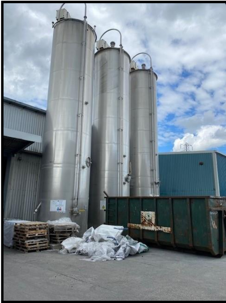
Photo 3 – Storage silos not yet commissioned.
