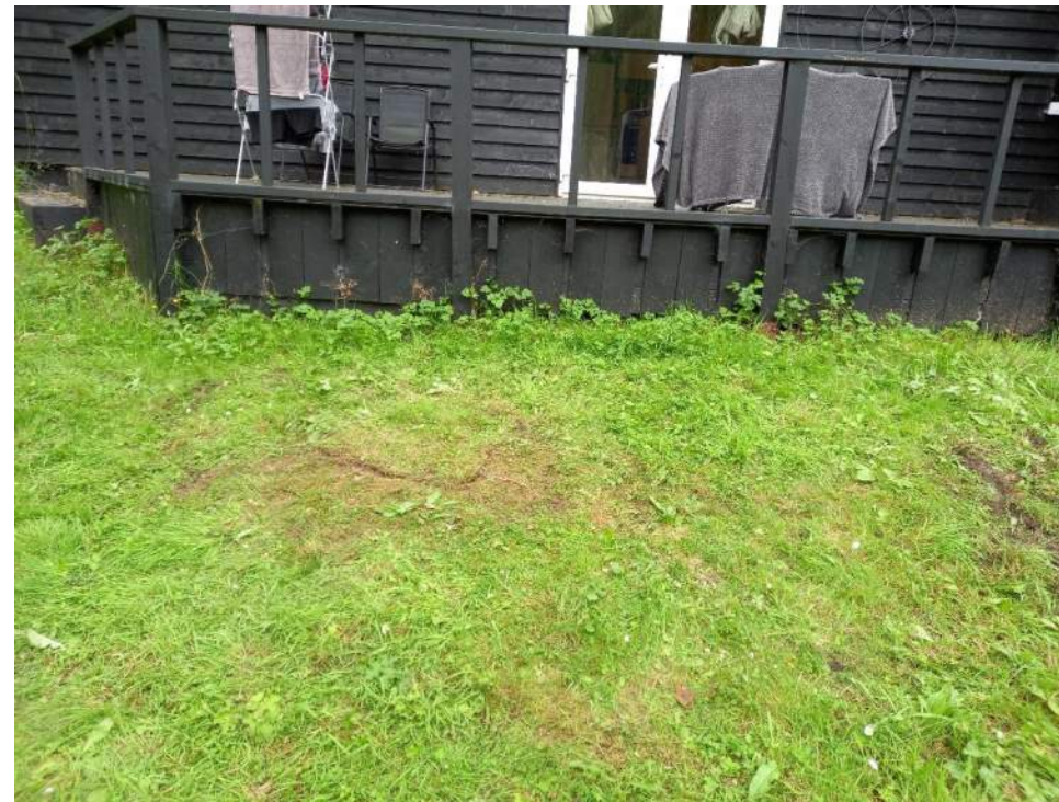
Photograph 8 – HP2 Post Condition
