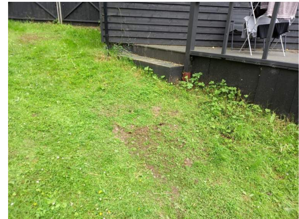
Photograph 12 – HP3 Post Condition
