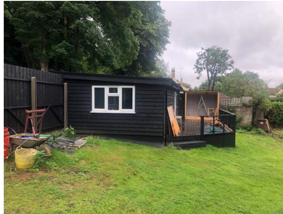
Photograph 2: View west of the site building
