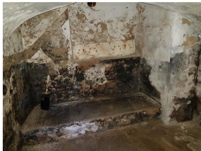
Figure 4: Barrell vault and cellar walls to be restored.
