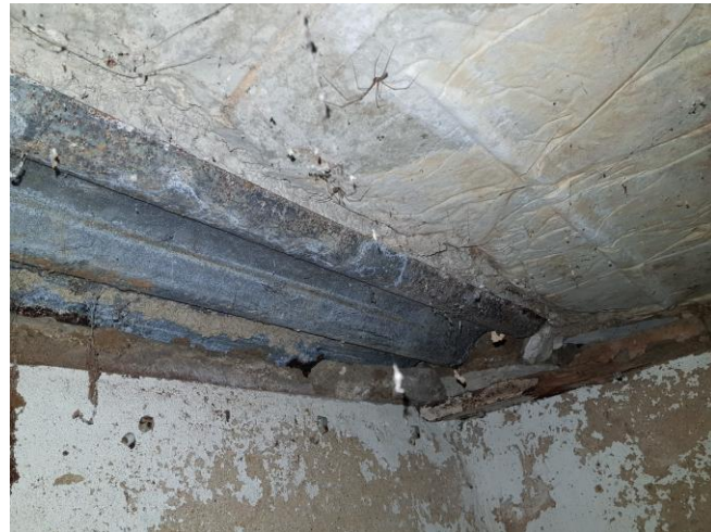
Figure 3: Internal access from the cellar to the living room has previously been filled in. The proposals seek to reinstate the access with the insertion of a spiral staircase.
