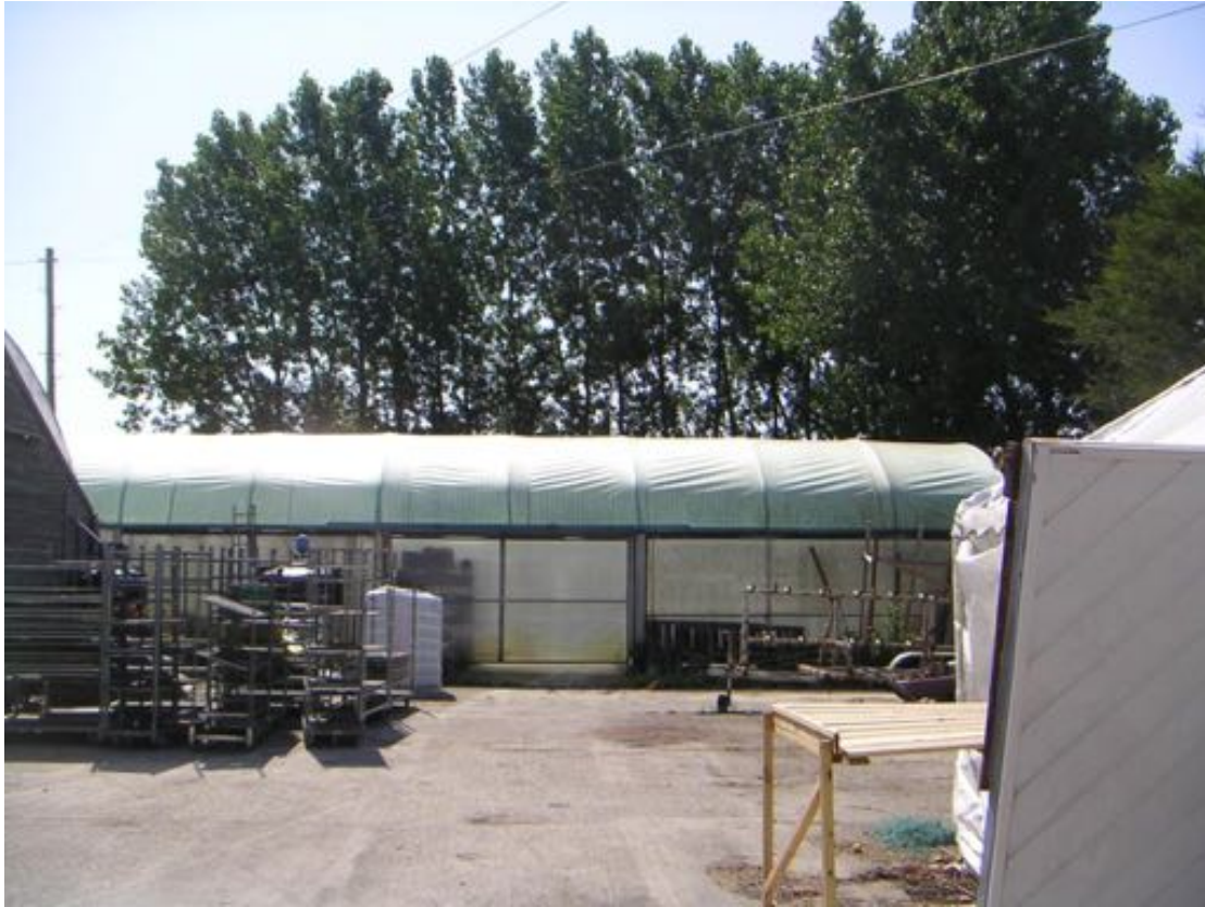
Photo 19 – Northern aspect of Building 11.
