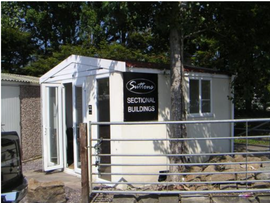
Photo 6 – Southern and eastern aspects of Building 5.
