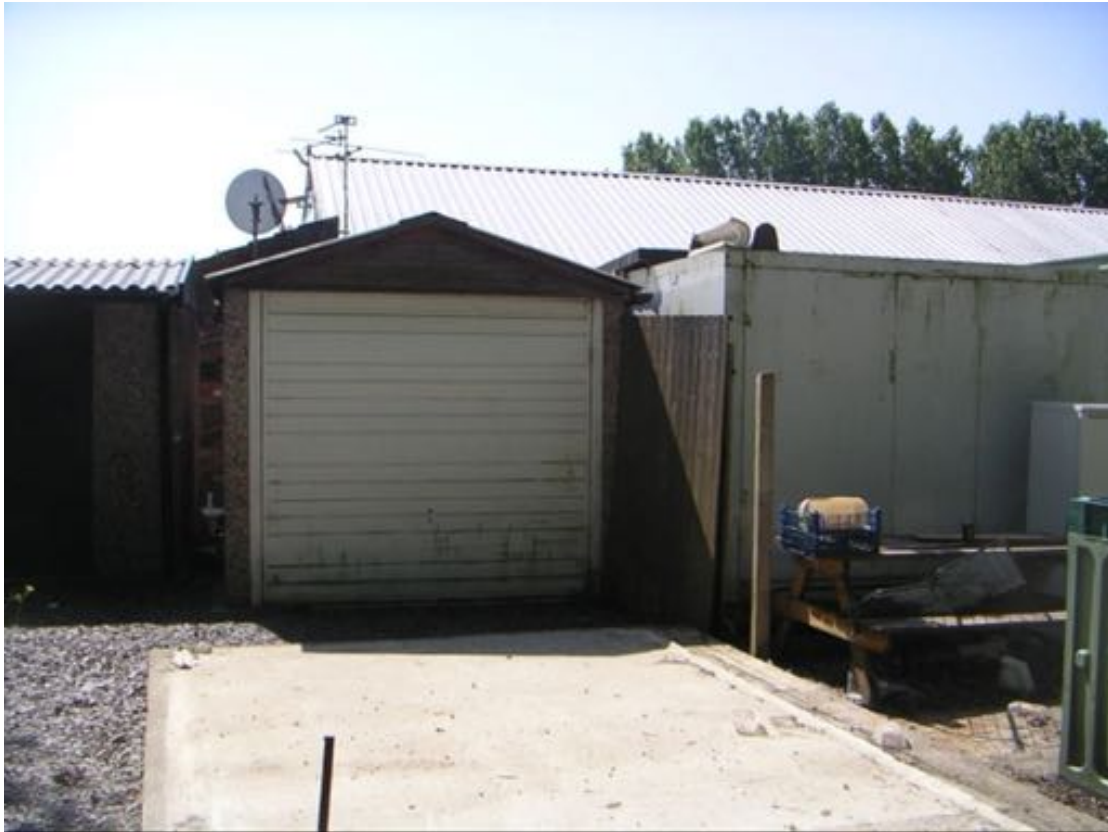
Photo 9 – Northern aspect of Building 8.
