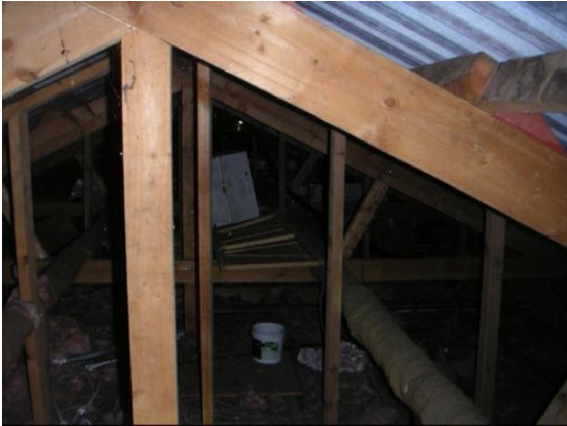
Photo 29 – Internal view of the northern section of Building 10.
