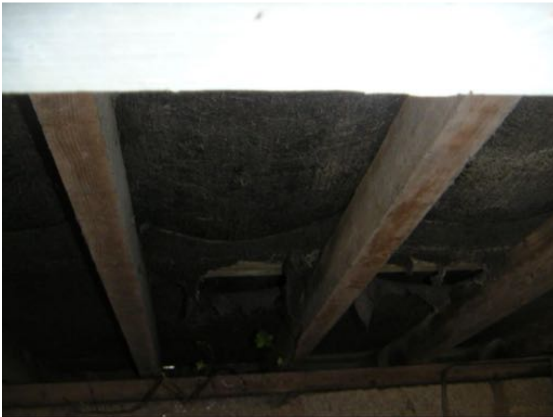
Photo 28 – Internal view of Building 2.
