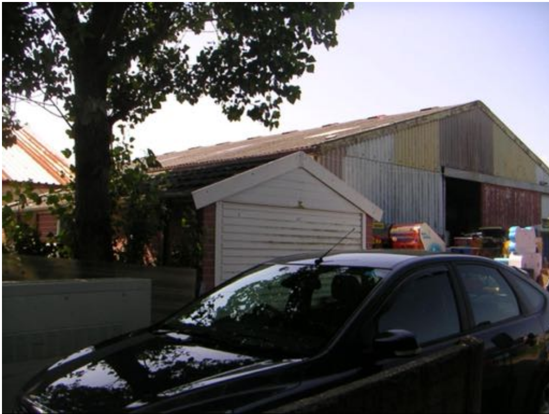
Photo 27 – Northern aspect of Building 16.
