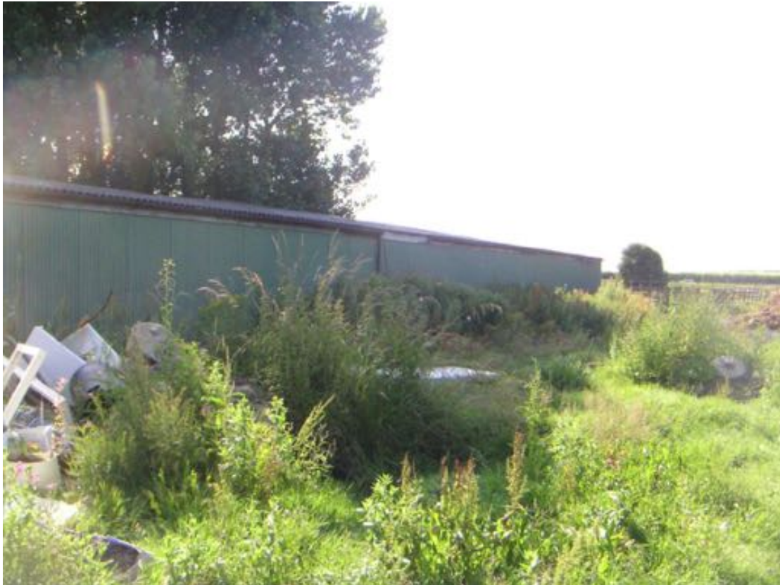
Photo 20 – Western aspect of Building 12.
