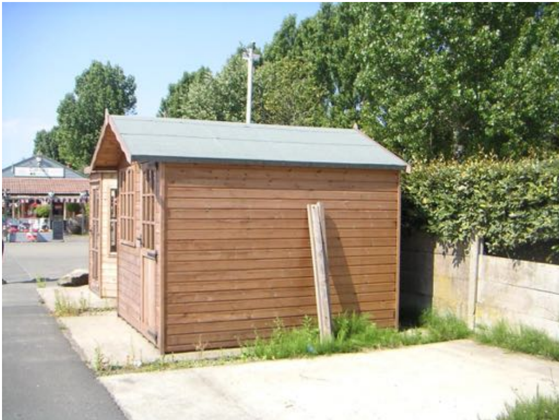
Photo 4 –Eastern aspect of Building 3.
