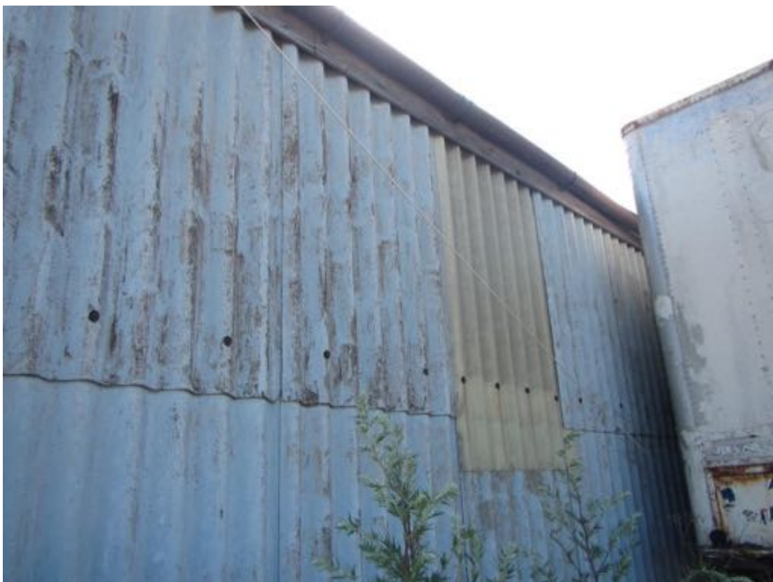
Photo 24 – Western aspect of Building 13.
