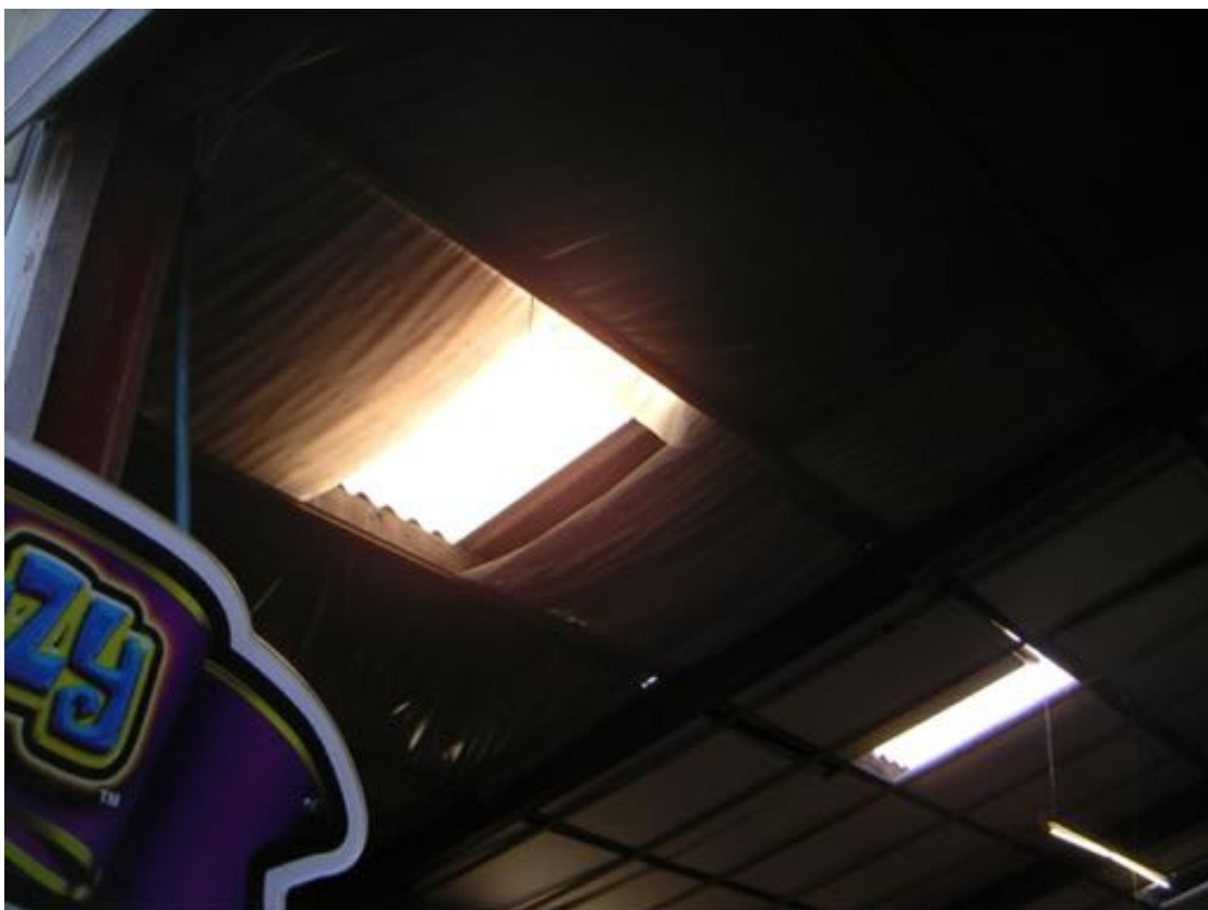
Photo 34 – Internal view of Building 13.
