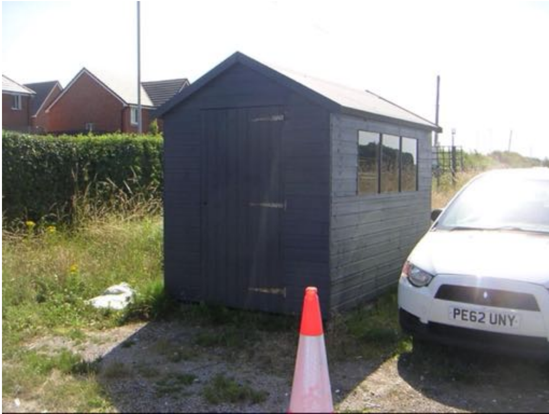
Photo 1 – Northern and western aspects of Building 1.
