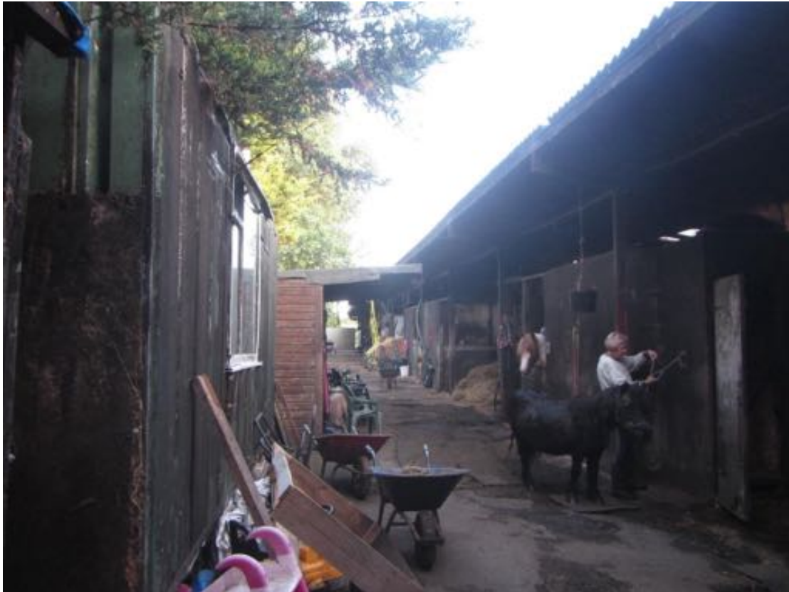
Photo 22 – Eastern aspect of Building 12, open fronted stables.
