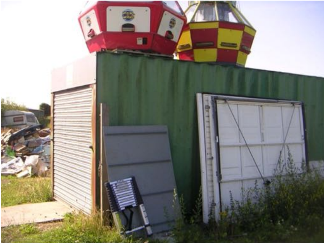
Photo 26 – Building 15, located immediately adjacent to the western site boundary.
