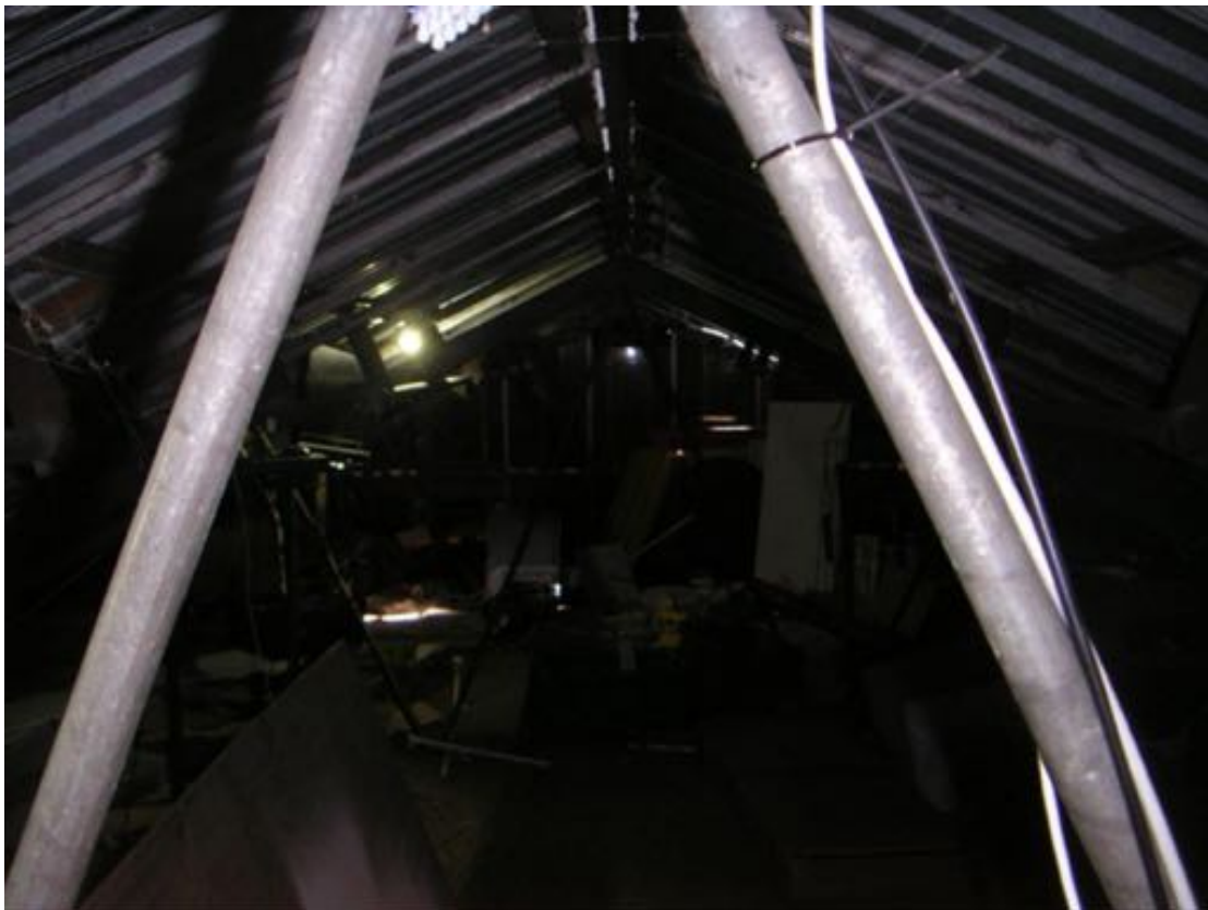
Photo 32 – Internal view of southern section of Building 10.
