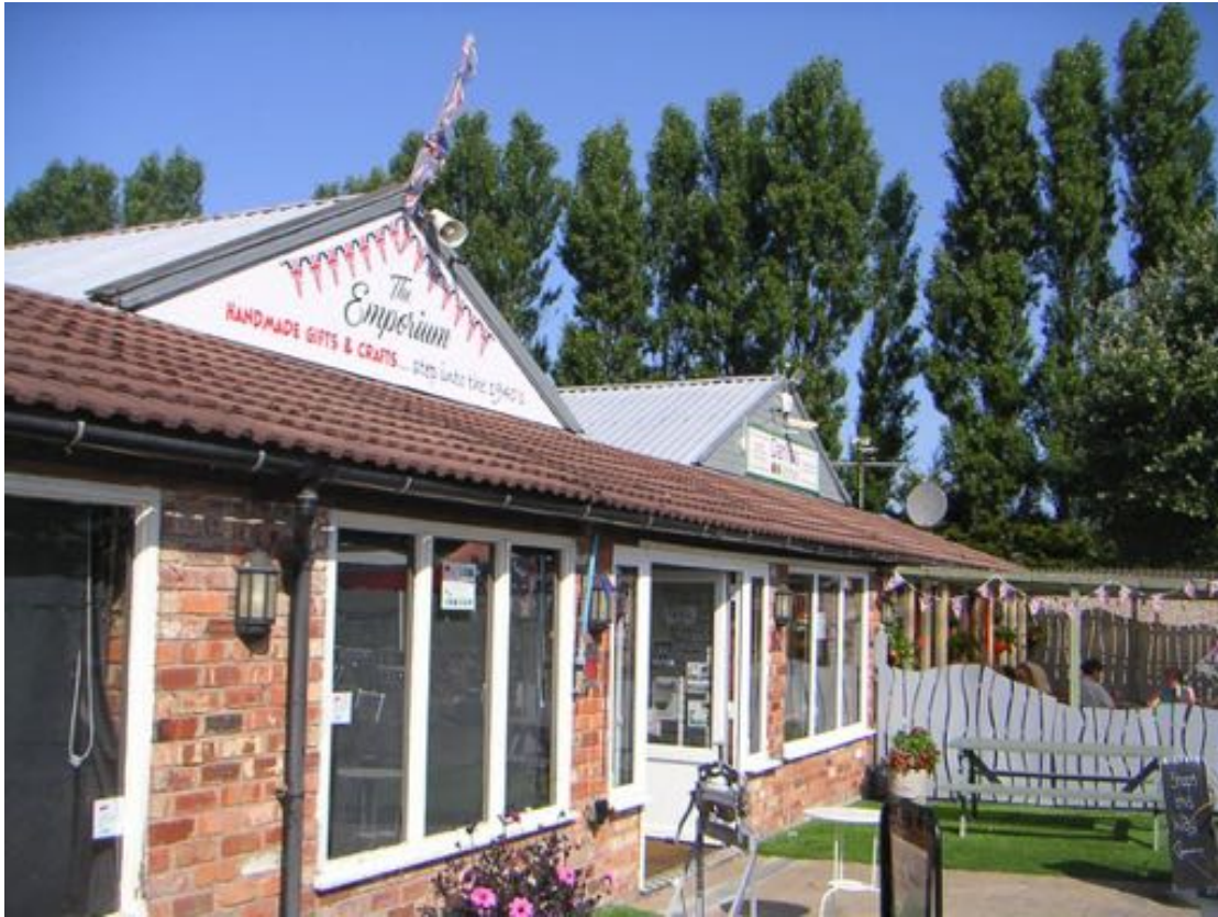
Photo 15 – Eastern aspect of Building 10.
