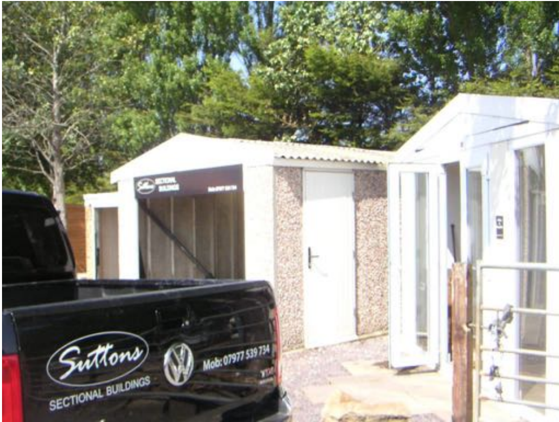
Photo 7 – Southern aspects of Building 5, 6 and 7.
