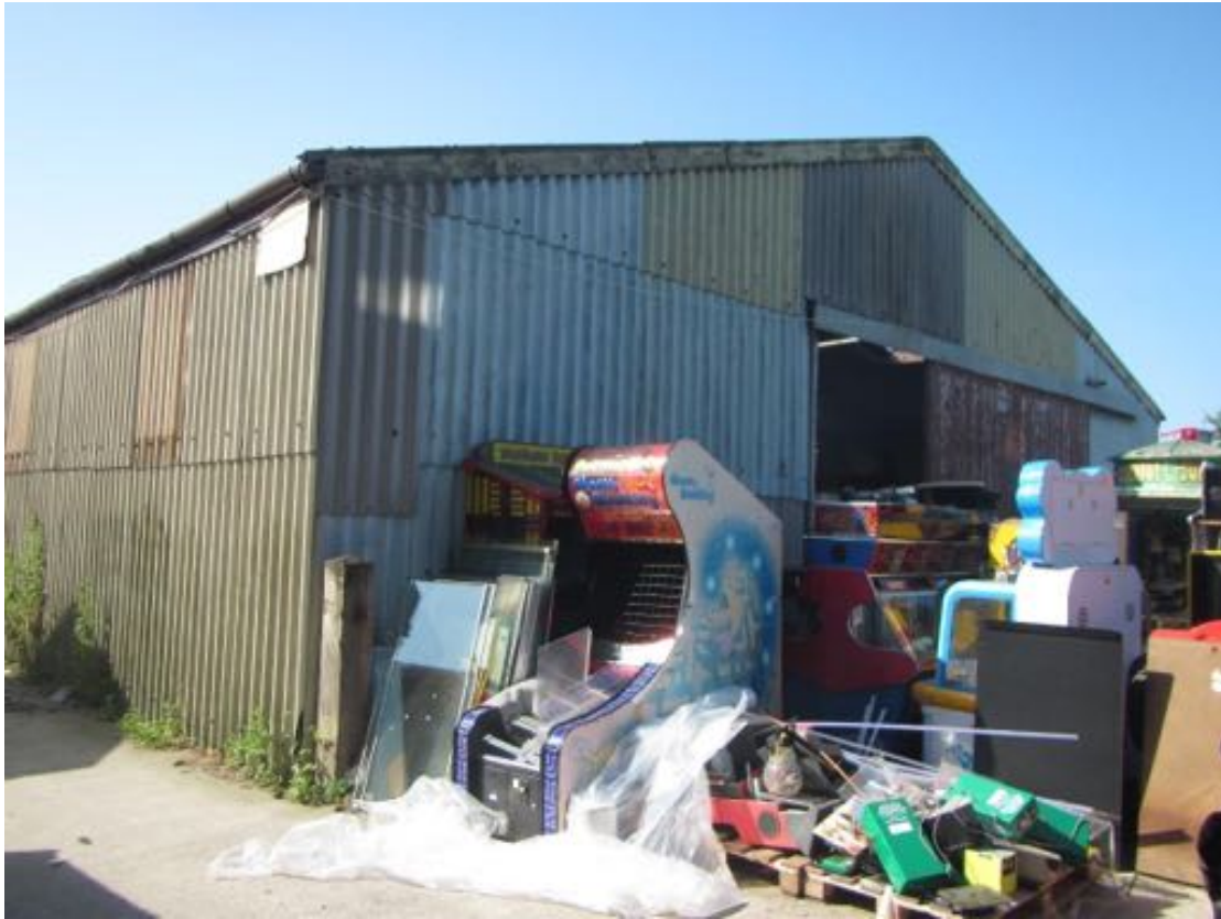
Photo 23 – Northern aspect of Building 13.
