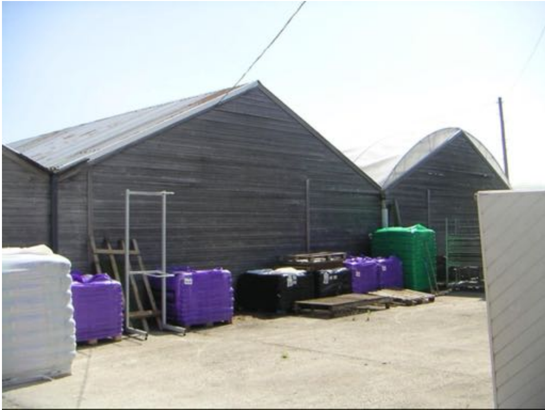
Photo 17 – Western aspect of Building 10.
