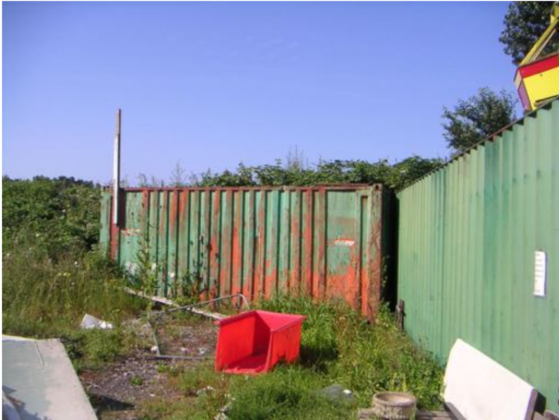
Photo 25 – Building 14, located immediately adjacent to the western site boundary.
