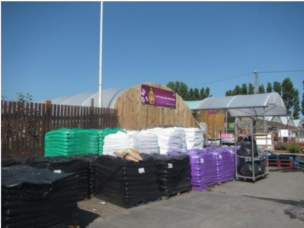
Photo 18 – Eastern aspect of Building 11.
