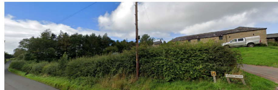
image of existing house + barns from public highway at drive entrance
