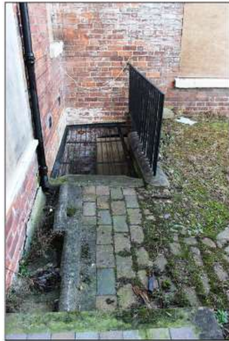
Plate 13 above: Cellar entrance below later 19 th century wing; not currently accessible
