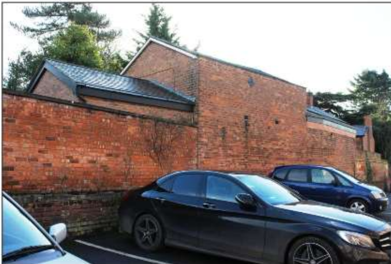
Plate 39: The Stables west elevation
