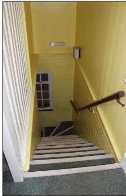
Plate 28 above: 1960s staircase
