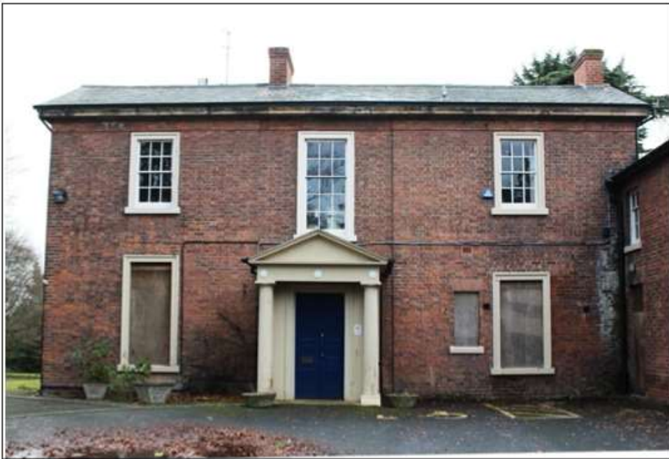
Plate 2 below: Chaddeslode House main / north elevation
