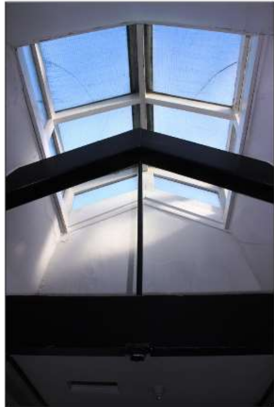
Plate 31: c.1840 north wing; renewed truss with bolted king-post below the skylight
