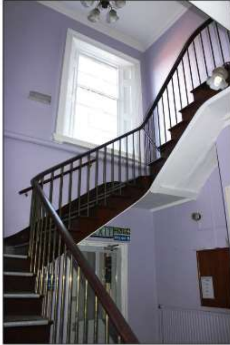
Plates 18-20: Main staircase to be retained in House B
