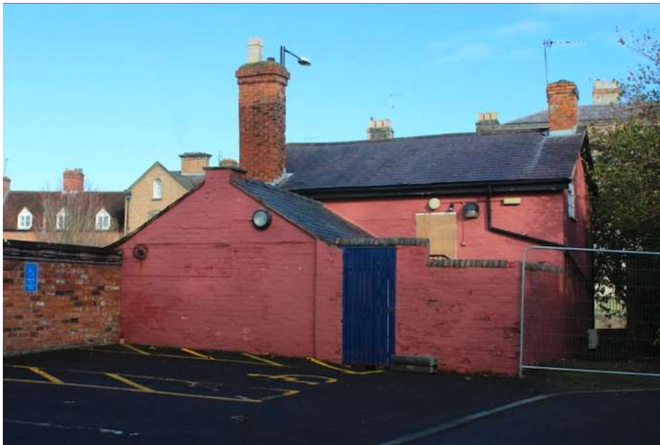
This was the cottage prior to the extensions above and below
