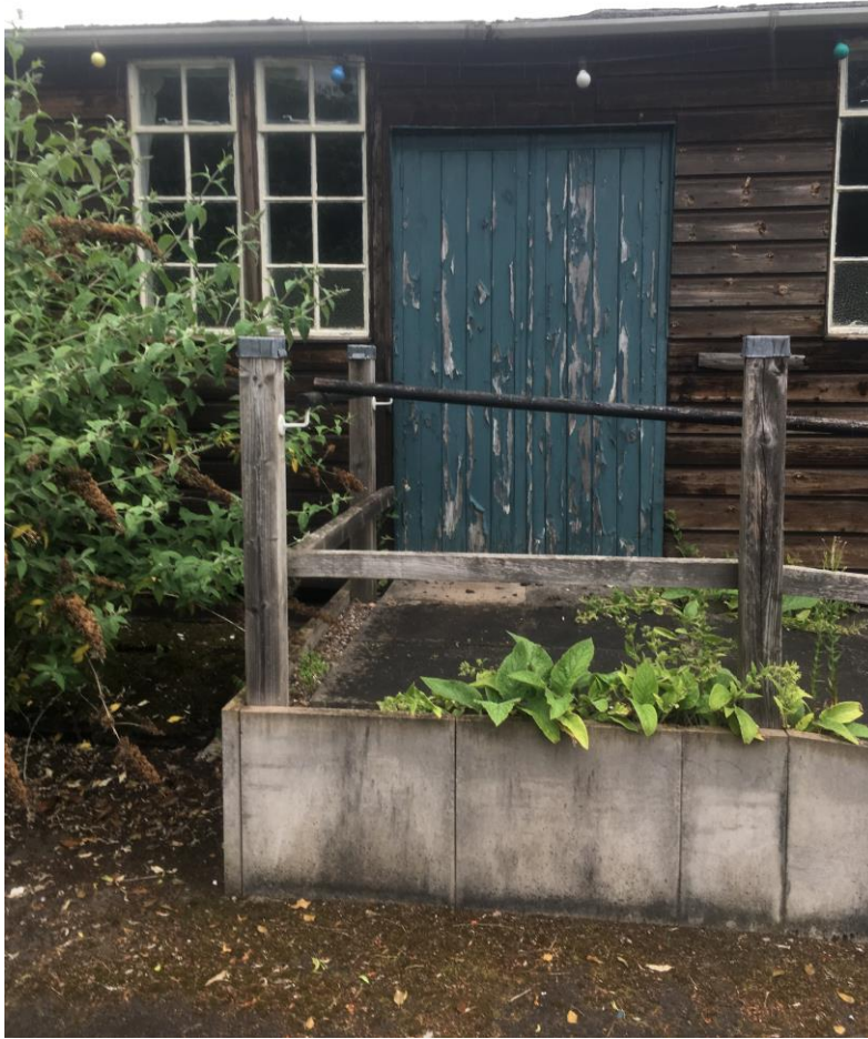
View of ramp to be retained
