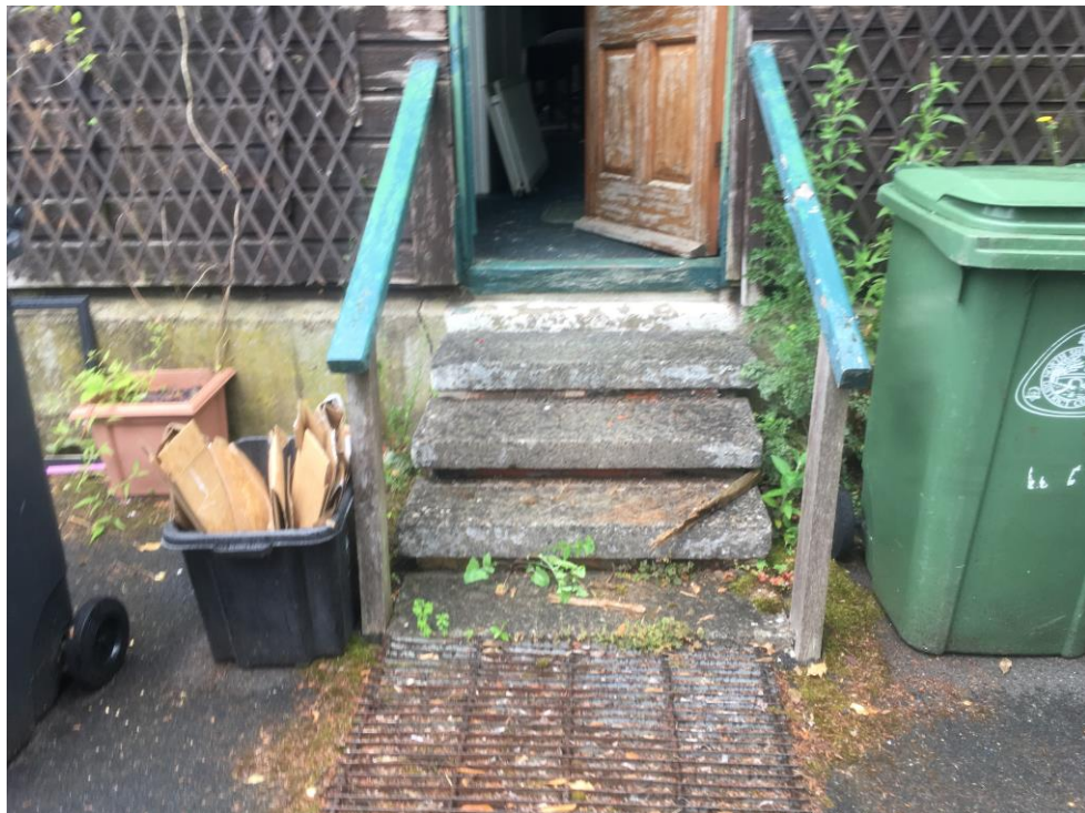
Steps to remain, handrails removed
