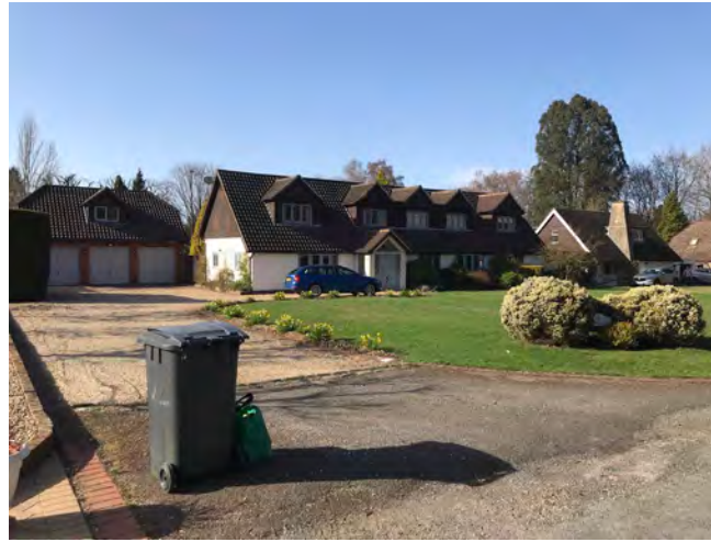
6 South Road – Neighbour to south west
