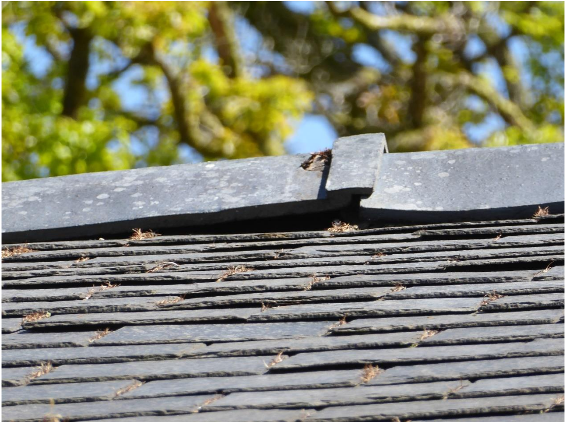
Photo's 7 & 8. Potential roost features were located under raised ridge tiles (above) and where boxed soffits had come adrift (below).
