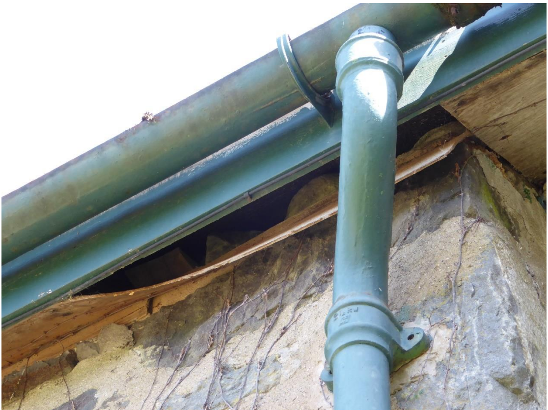
Photo's 7 & 8. Potential roost features were located under raised ridge tiles (above) and where boxed soffits had come adrift (below).
