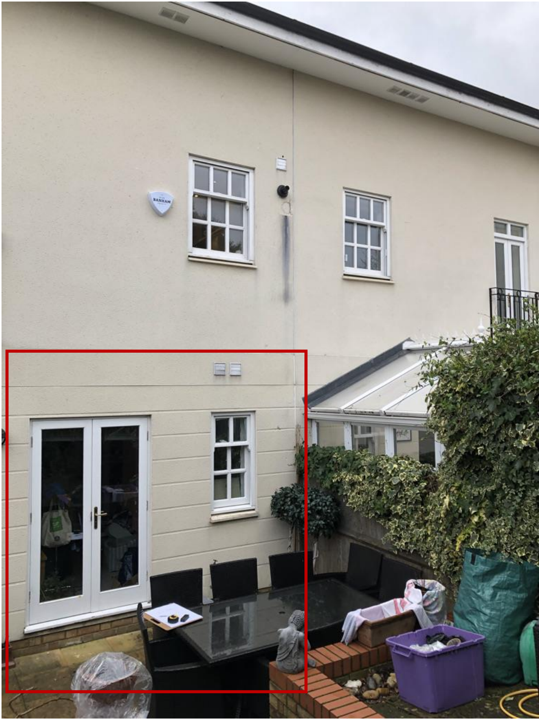
Rear Elevation (North) View from public private garden Location of proposed extension
