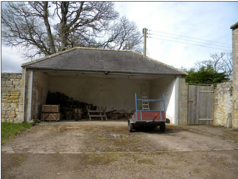
Figure 29. Garage (southern elevation), open access.
