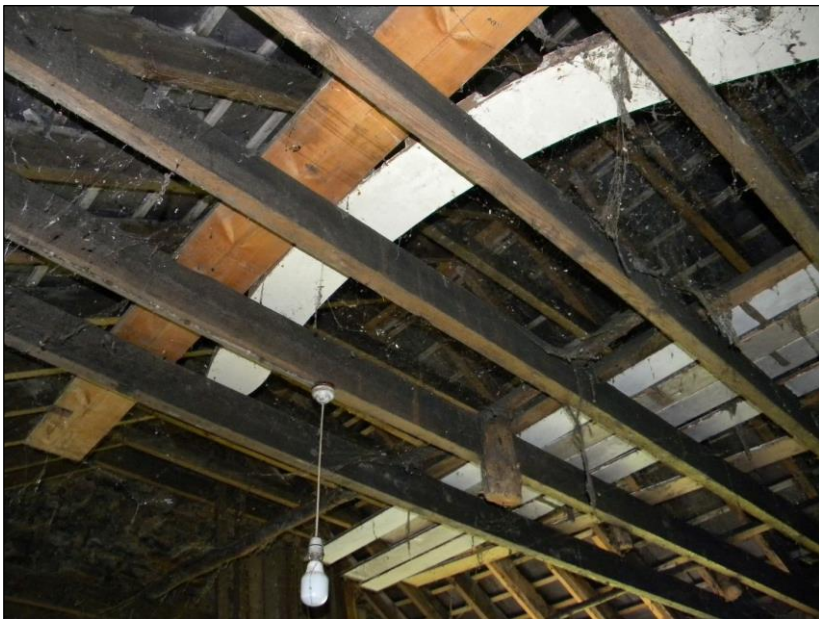
Figure 35. Cartshed open roof to pitch – lots of cobwebs.
