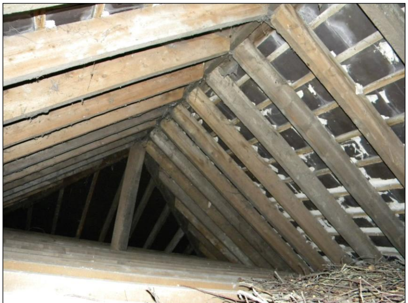
Figure 30. Roof structure within garage loft void – swallows and jackdaw nests.
