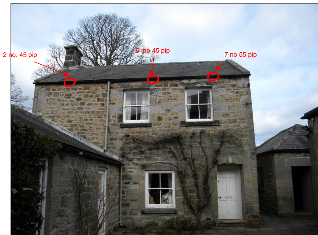
Figure 46. Bat roost locations within the cottage (front elevation).
