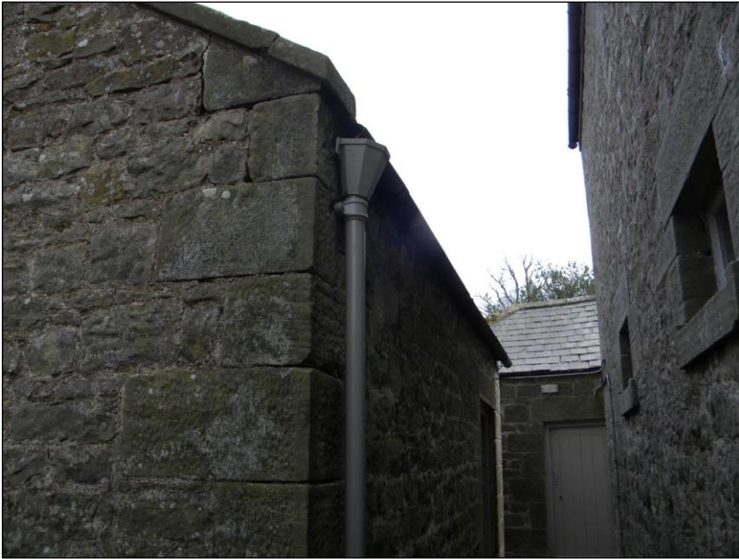
Figure 37. Cartshed south west elevation adjacent to cottage (area affected by works).
