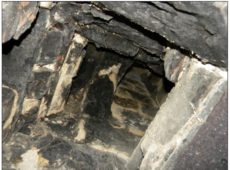
Figure 20. Chimney above range on upper floor in stables.
