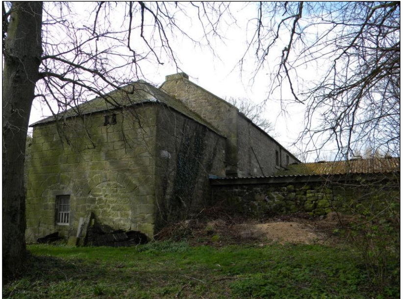
Figure 11. Rogue external end gable of dovecote and rear elevation of stables.
