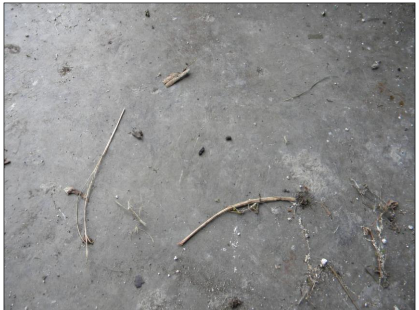
Figure 36. Bat droppings within cartshed.
