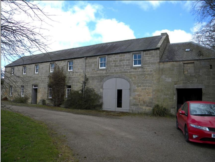
Figure 10. South west (front) elevation of stables showing dovecote to the right.
