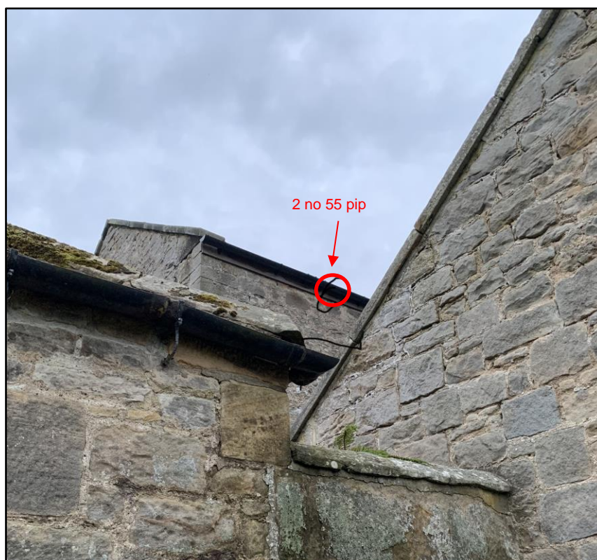
Figure 47. Bat roost locations within the cottage (rear elevation).
