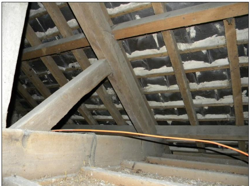
Figure 24. Internals of loft above stables.
