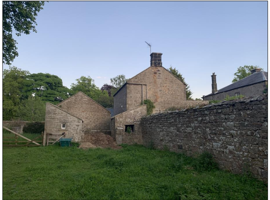
Figure 40. Rear of cottage. North west elevation.
