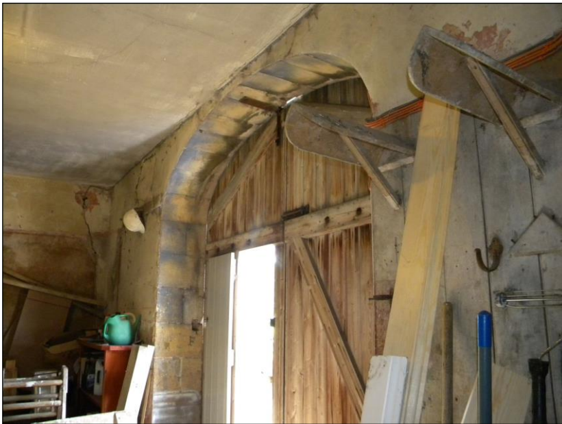
Figure 17. Archway access to lower floor of the stables.
