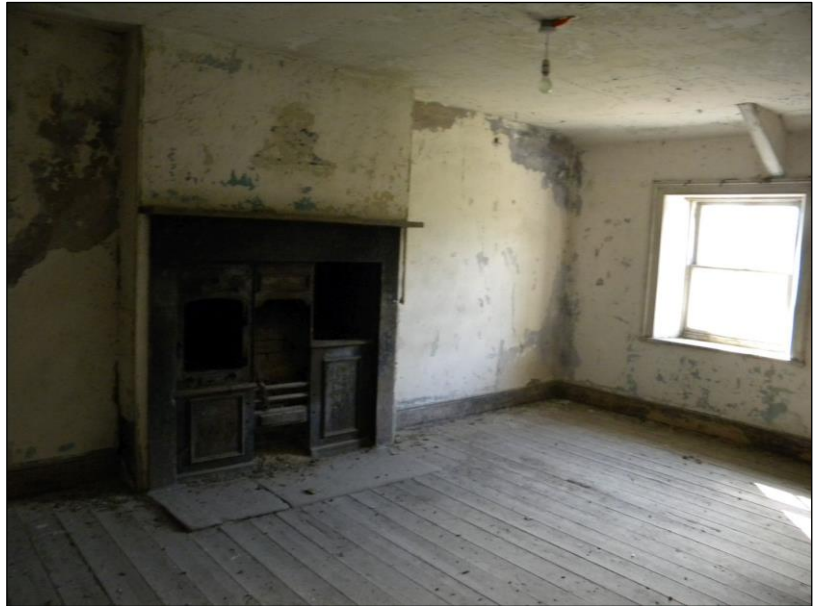
Figure 22. Upper floor room above stables.
