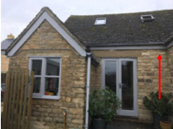
Photograph 1: Roost location on north-eastern elevation
