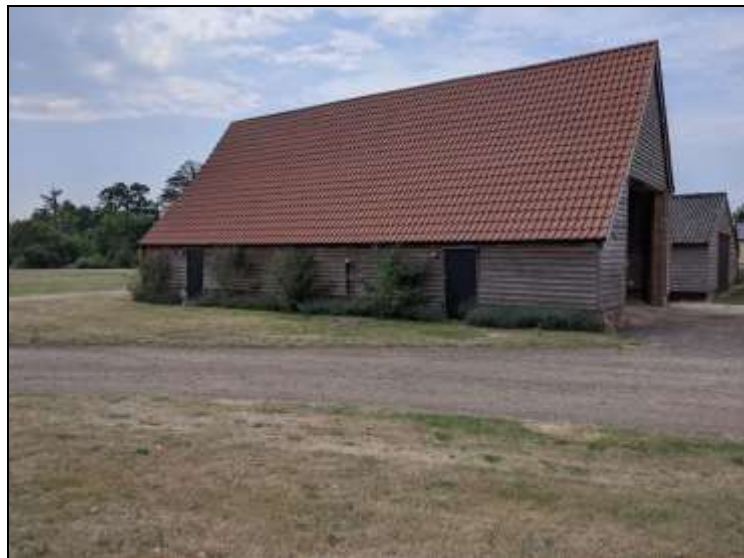
Figure 2.8 Barn to the west
