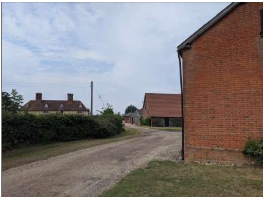
Figure 6.2 View of Rockylls Hall from the Application Site
