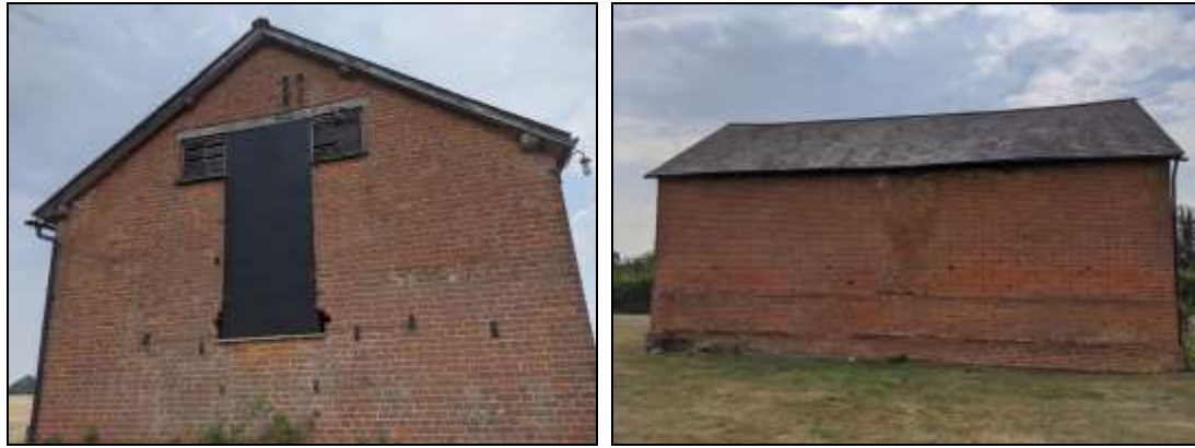
Figure 2.5 North western and north eastern elevations
