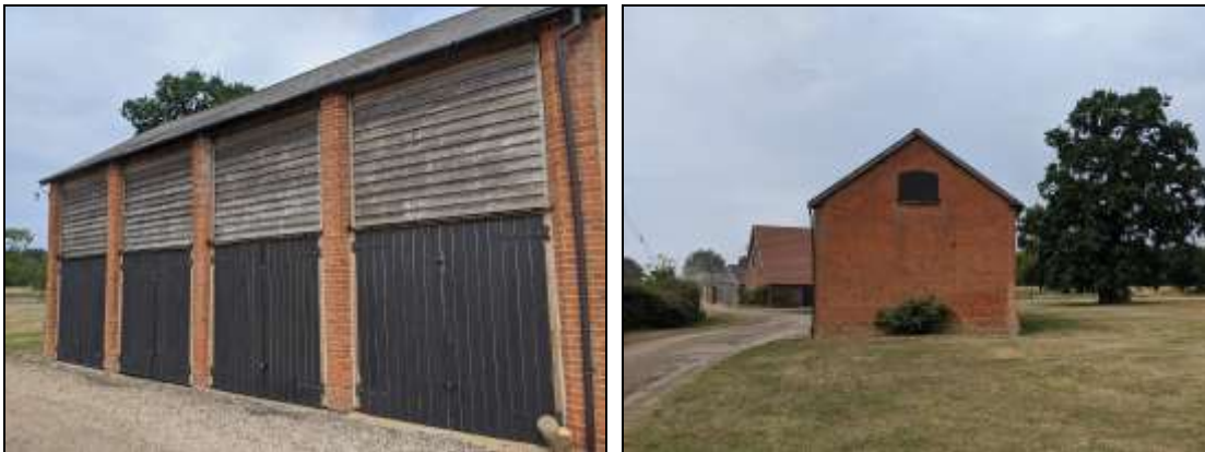
Figure 2.4 South western and south eastern elevations
