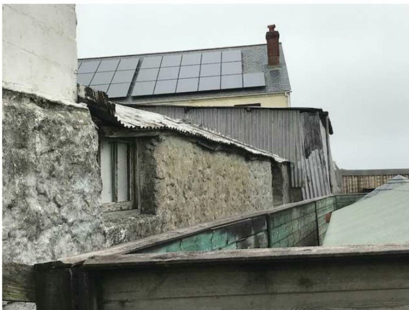
Figure 3: View of south elevation of the old piggery.
