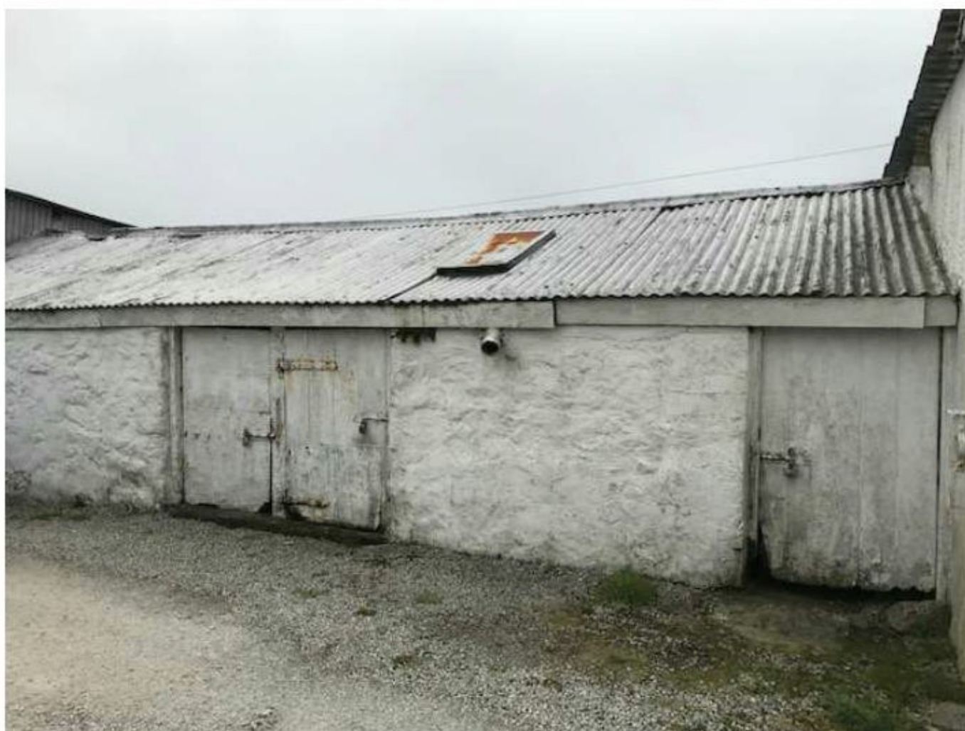
Figure 1: View of north elevation of the old piggery.
