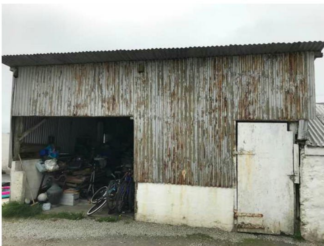
Figure 2: View of north elevation of garage.
