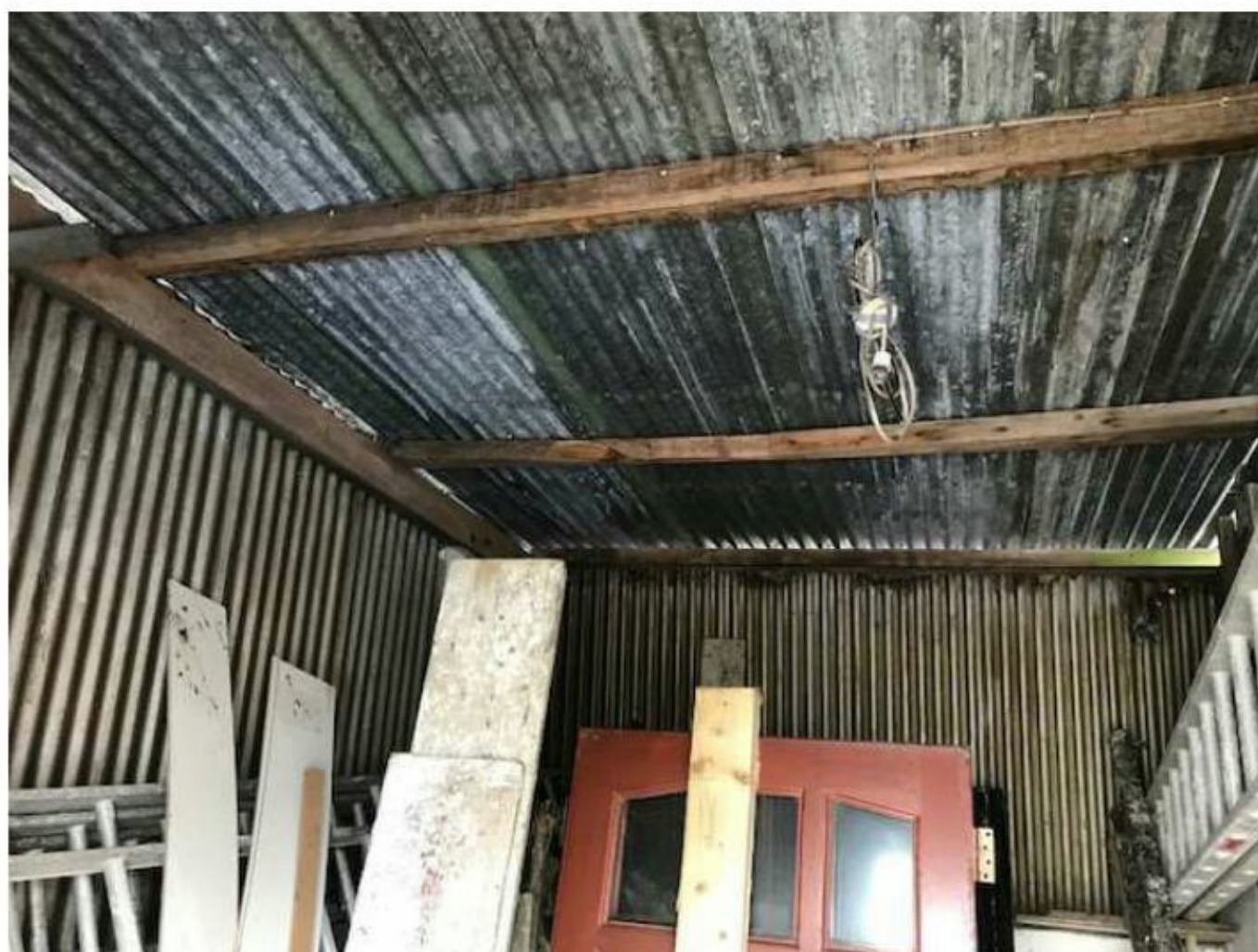
Figure 5: View of interior of garage.
