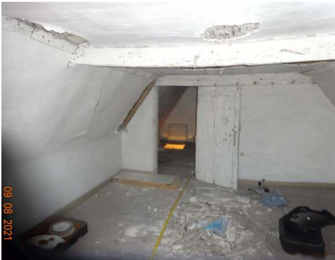
Photograph showing the current condition of the Second Floor.
