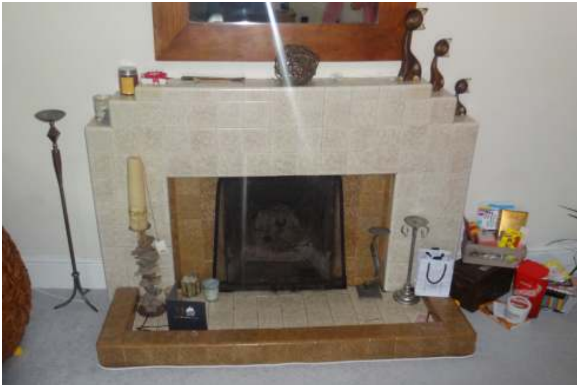
Photograph showing the existing lounge fireplace
