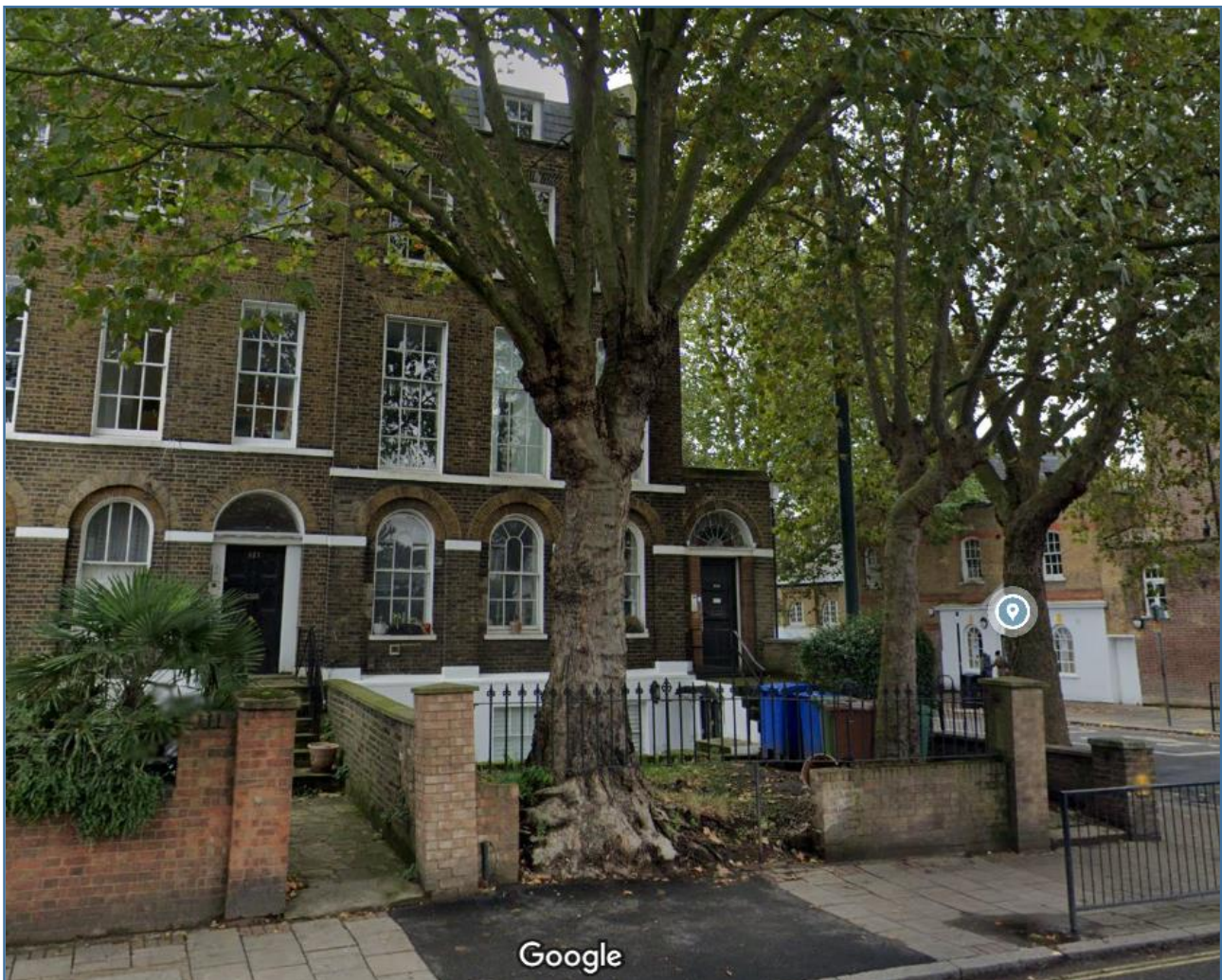
FIGURE 1 - PHOTO OF SITE FROM STREET VIEW
