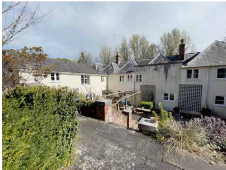
2. North Side: Site of Staircase Extension
