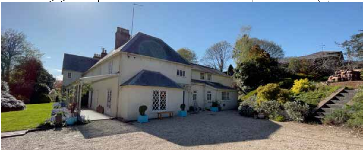
Current Photo from the driveway - looking north west
