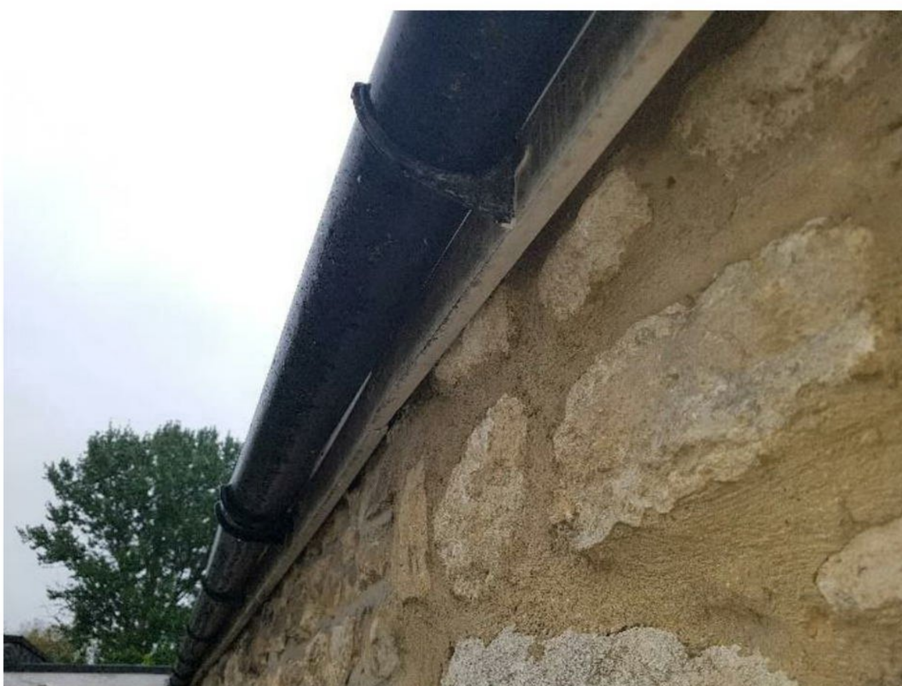
Photograph 3. 19 Gaps beneath weatherboarding on the northern face of the dwelling.
