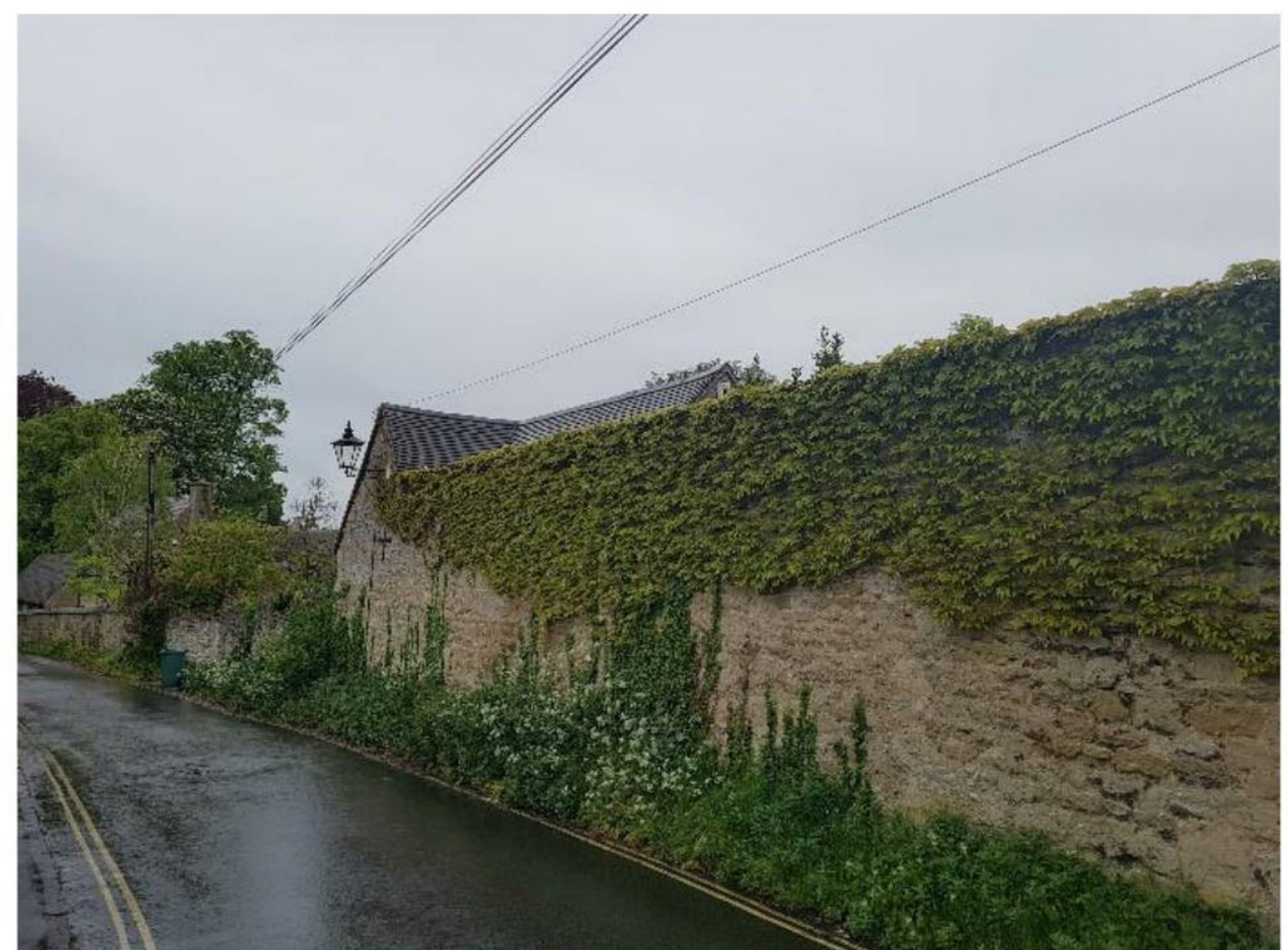
Photograph 6. The western ruin wall viewed from the south-west.
