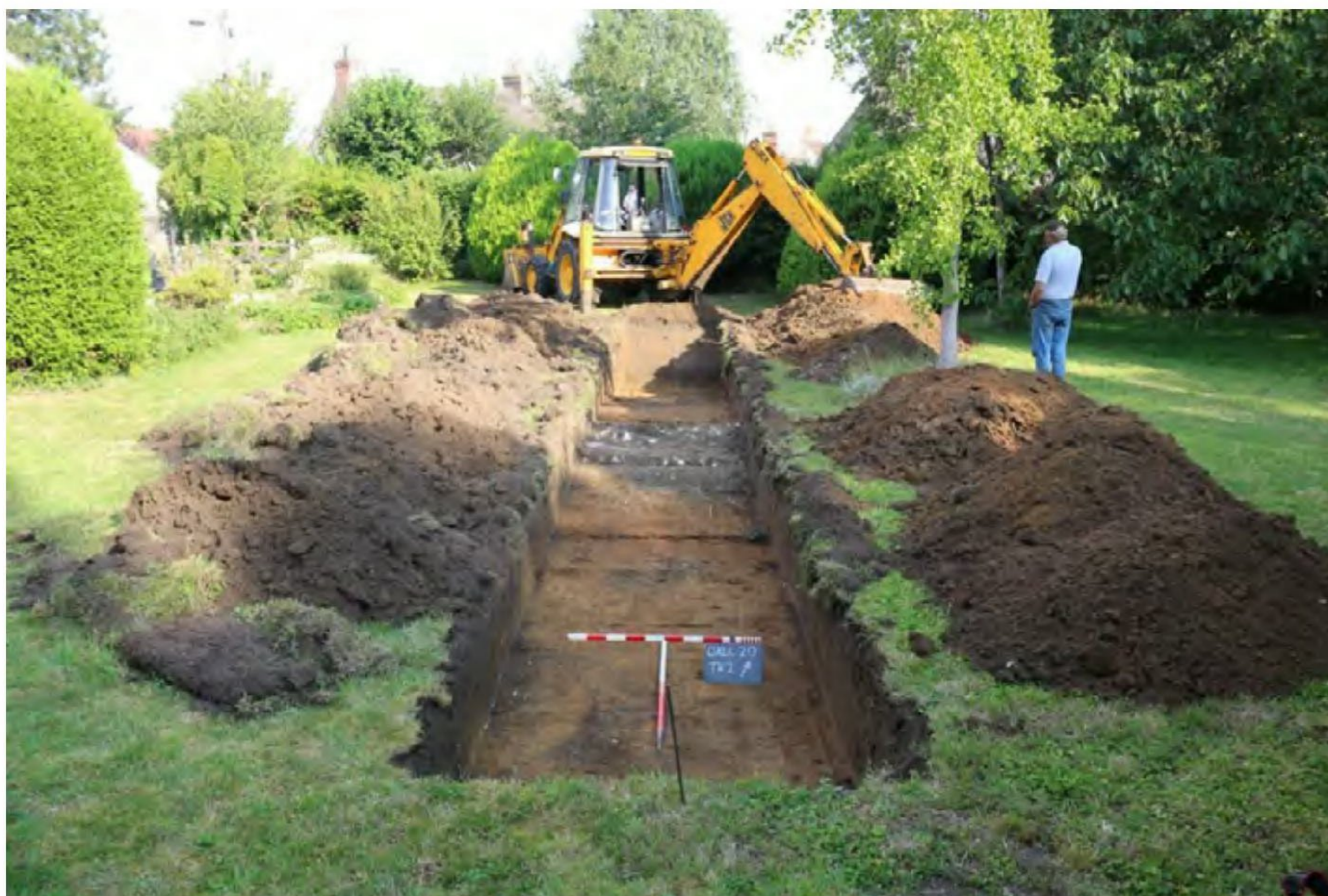
Plate 2: Trench 2, pre-excavation. Looking north
