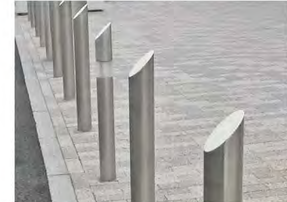
Stainless steel bollards used to restrict vehicular access to plaza
