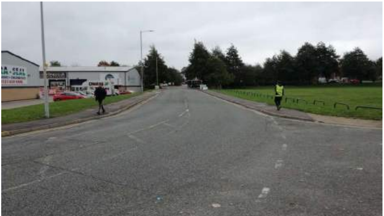
Photograph 3.3: Welton Road (east) - southbound
